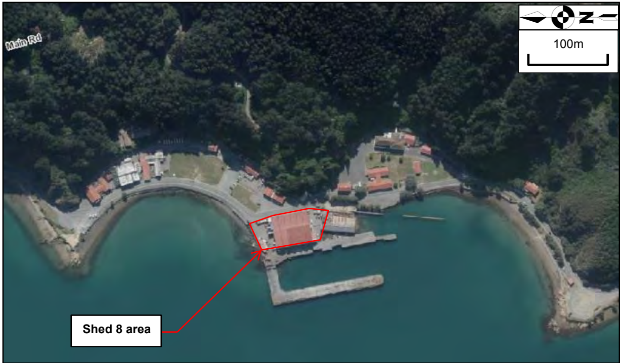
Figure 1 Aerial Photograph, Shelly Bay, 2013 (Ref. 4)
