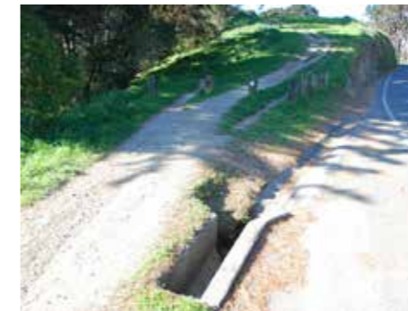
5. Trip and Fall Hazards
