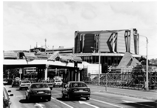
Landmark structures on entrance routes
