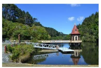
**Figure 8.** The Karori Reservoir Tower houses the valves that were originally used to control water levels in the Karori Dam. It is now part of the Zealandia Wildlife Sanctuary, and part of the story of water supply infrastructure in Wellington. (Photo: Wellington City Council, 2015)
