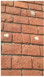
**Figure 39.** The façade at 15 Tory Street has been secured with concealed fixings. The holes have been filled, and coloured to match the existing brickwork. (Photos: Wellington City Council, 2018)
