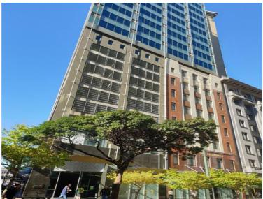
**Figure 35.** Façadism (or façade retention) is the preservation of the exterior face/faces of a building without the three-dimensional built form providing for its structural support and understanding of its function.
