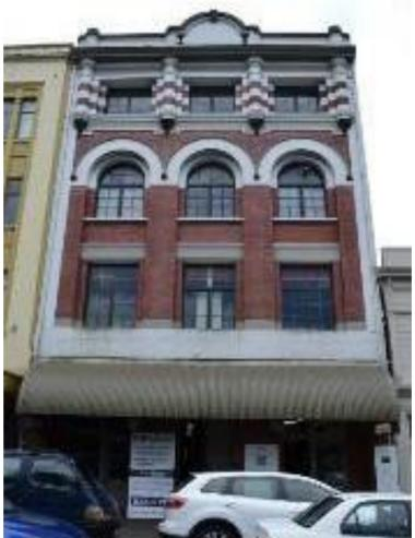
**Figure 38.** The former Cadbury's Building at 60 Ghuznee Street, Wellington was strengthened in 2017. There are new internal reinforced concrete columns, steel cross bracing, and concealed stainless steel in the decorative columns on ground and third floors. The parapet has been restrained by a steel frame that is fixed back to the existing structure.
