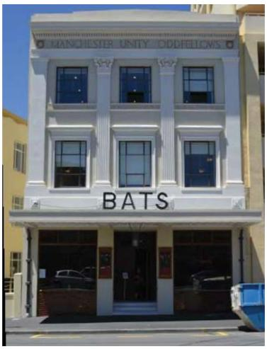
**Figure 37.** Bats Theatre at 1 Kent Terrace was strengthened in 2012 with new internal reinforced concrete columns and shear walls. There are new internal columns at the front elevation that continue from ground to roof level and support the parapet and façade. These have been designed so that they do not alter the street façade of the building.
