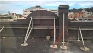
**Figure 42.** New structural elements to secure the existing parapet and chimney at the former Cadbury Building has been installed so that it is not visible from Ghuznee Street. (Photo: Wellington City Council, 2018)
