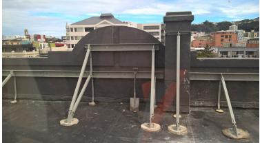
**Figure 42.** New structural elements to secure the existing parapet and chimney at the former Cadbury Building has been installed so that it is not visible from Ghuznee Street. (Photo: Wellington City Council, 2018)
