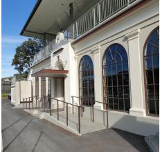
**Figure 47.** After - The non-heritage doors were replaced with new timber joinery to match the original drawings from 1924. The door leaves have been adjusted to meet requirements for accessibility. A second ramp has been added to make the entrance symmetrical, and the handrails updated. (Photos: Wellington City Council, 2020)
