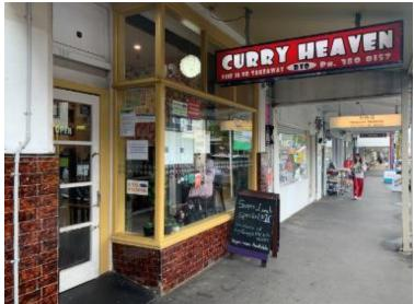
**Figure 17.** This shopfront in the Newtown Heritage Area has been restored by careful work to uncover and make good the original shopfront. Paint was removed from the original tiles, a bulkhead was removed from the interior, and a replica window was constructed to the same dimensions and profiles. The shopfront restoration and structural strengthening have enhanced the heritage values of the Newtown Shopping Centre Heritage Area. (Photo: Wellington City Council, 2017)
