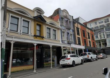
**Figure 12.** This well-considered redevelopment of an empty corner site has enhanced the Cuba Street Heritage Area. The heights of the parapet and verandah are consistent with the neighbouring heritage building. The ground floor shopfronts include traditional elements including recessed doors and shopfront display windows with tiled upstands. (Photo: Wellington City Council, 2020)
