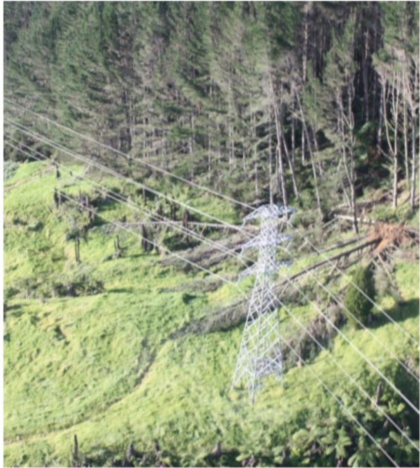
Photo 3: Northland tree fall example on Henderson-Maungatapere A 110kV transmission line
