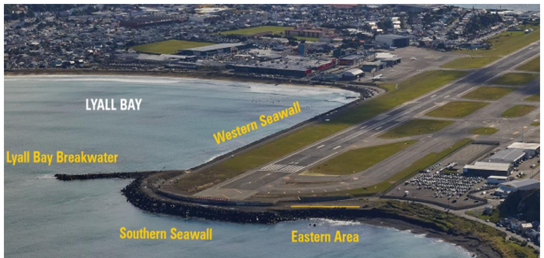
Figure 1: Seawall Structures Lyall Bay
