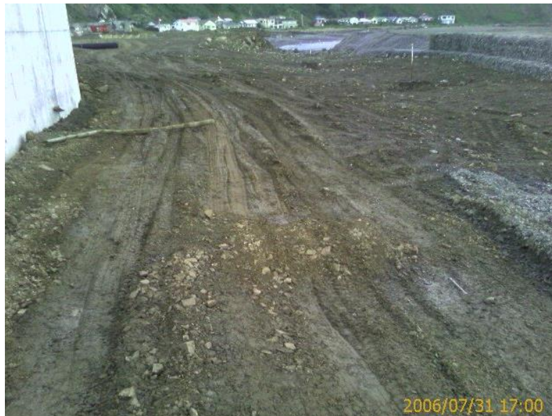
Photo N: During construction of RESA tunnel 2006 (WIAL files)
