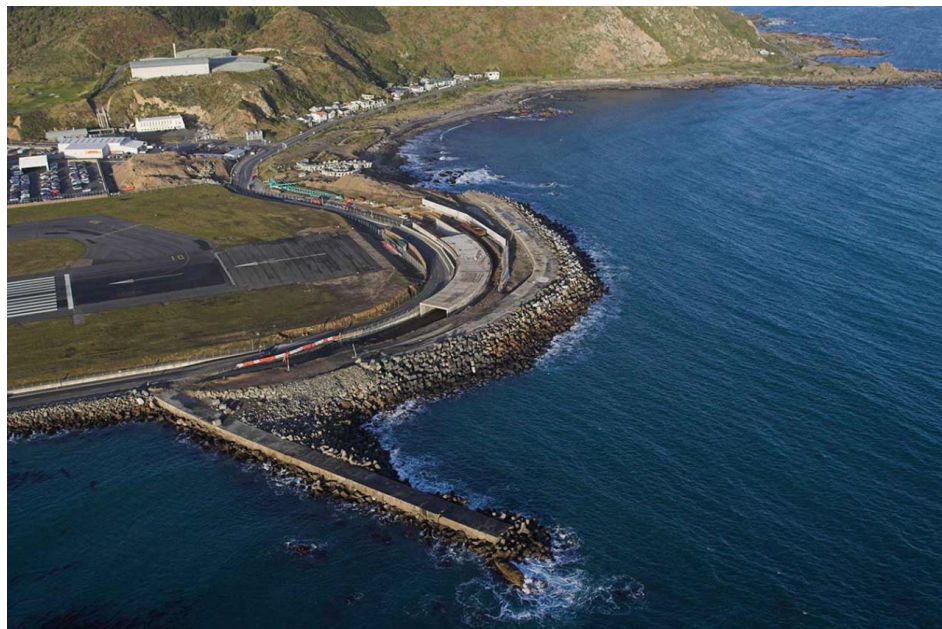
Photo O: 2006 construction of the RESA tunnel (WIAL files)
