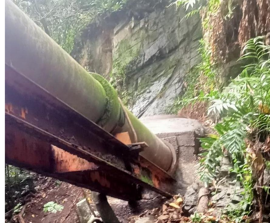
The waste water pipe has a high risk rating in the Wellington Water(WW), operational risk register and has been highlighted to WW Service planning as *in the event of failure it is unlikely that the pipeline will be able to be repaired, reconstructed or rehabilitated in the existing location due to safe access.*
