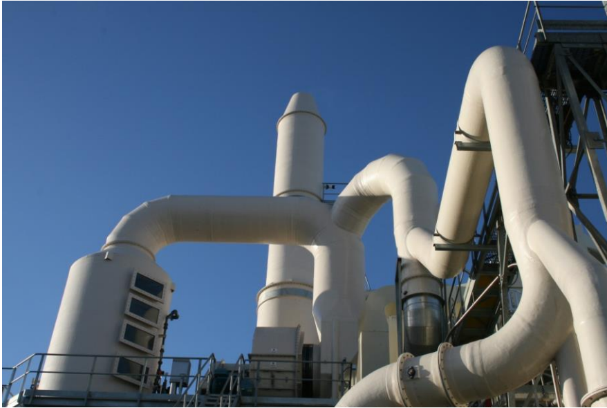
Photo 6: Air abatement system featuring air collection ducting, scrubber to remove particulate and odour, fan to move air, and stack for final dispersion
