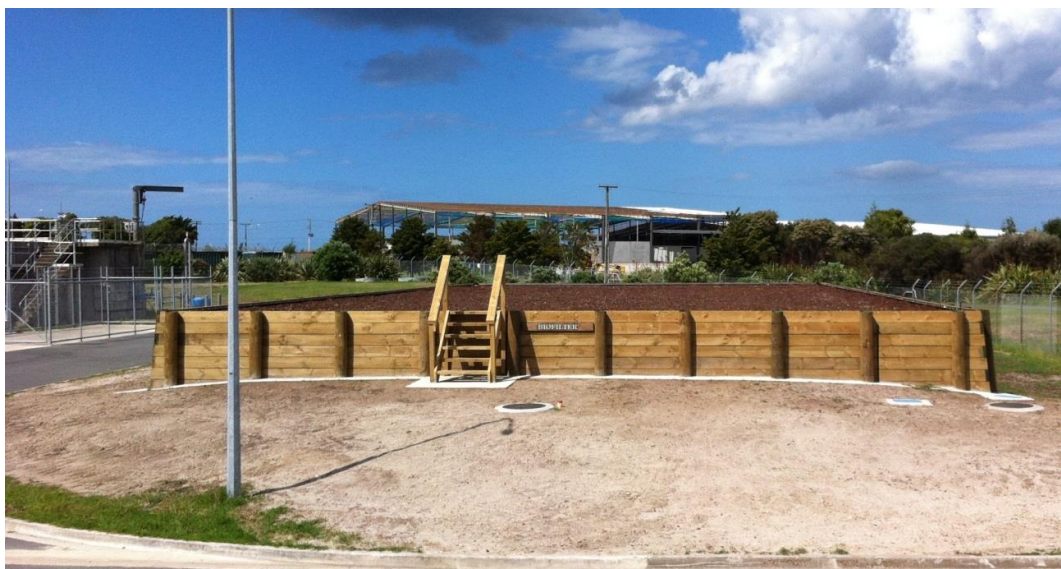
Photo 4: Biofilter at a wastewater treatment plant
