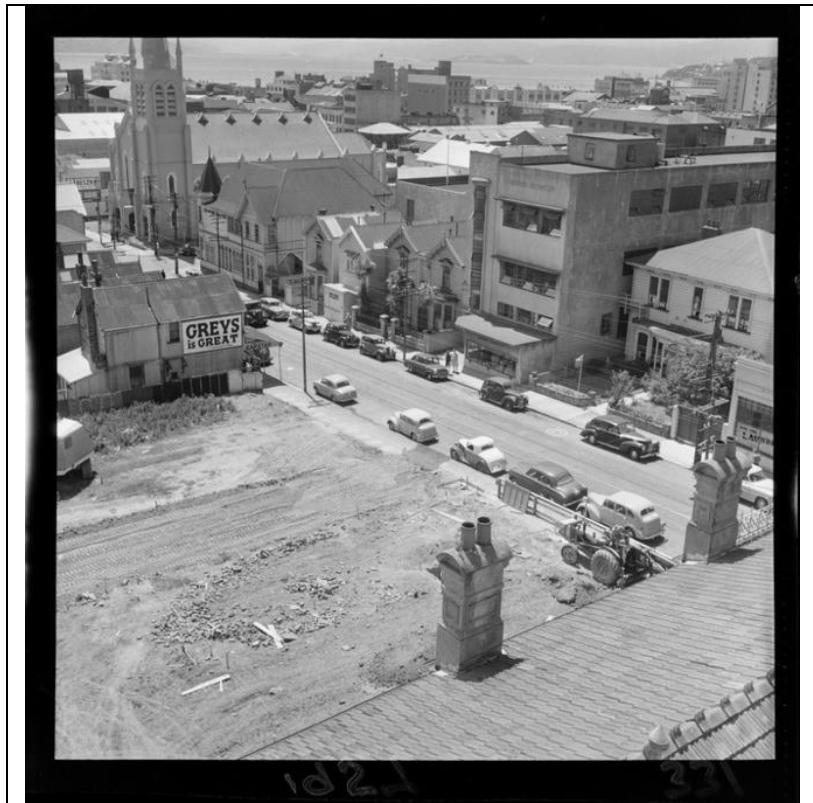
Image 3: (1957) Streetscape 233 Willis Street (Source Archives New Zealand). The building is an example of the open factory design model incorporating bands of windows to let light and fresh air into the building for the workers.
