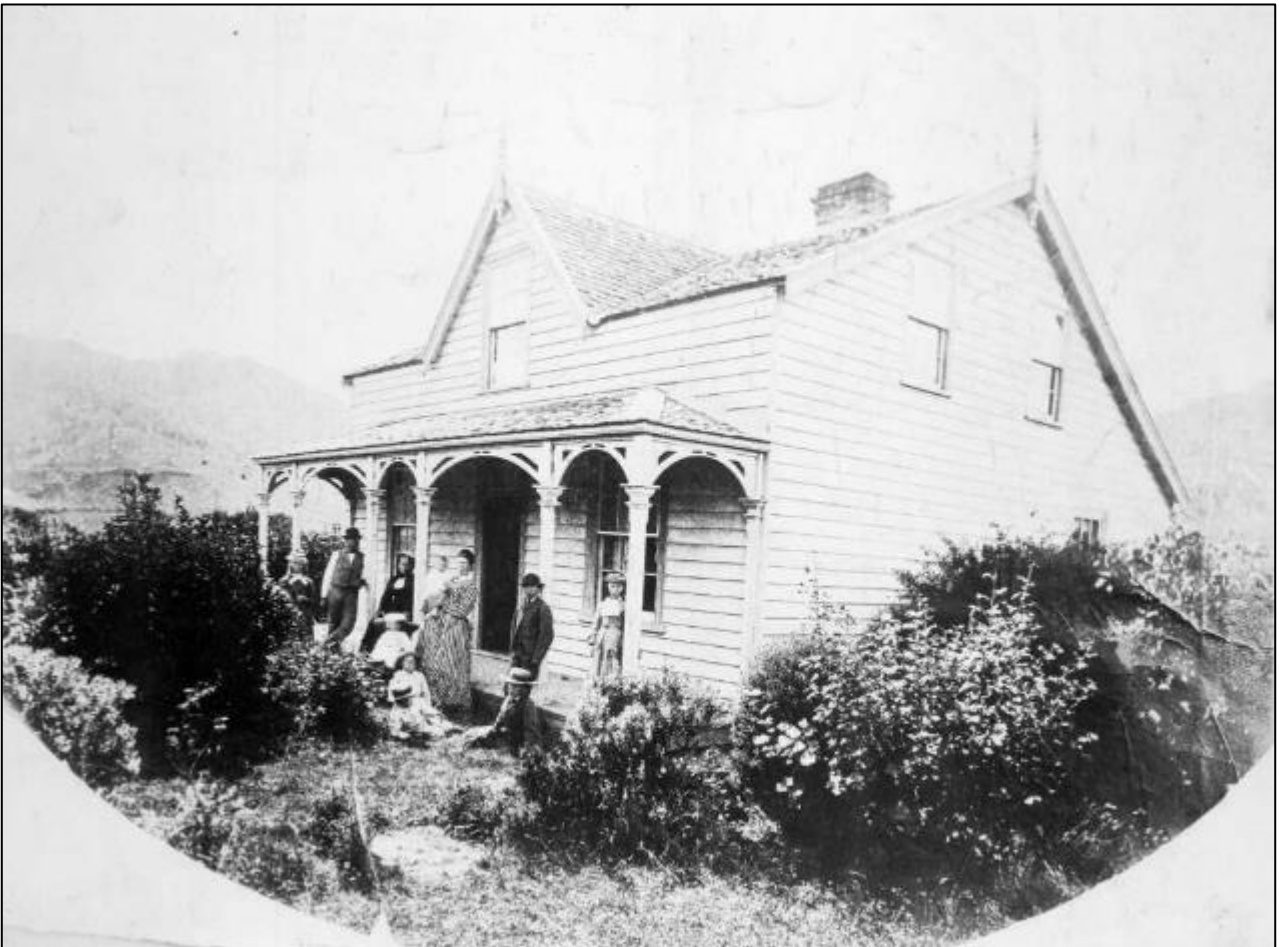
378 Karori Road, first home of Stephen Lancaster built in 1859. Note the similarity of architecture to Willow Grove (Unknown, 1860).
