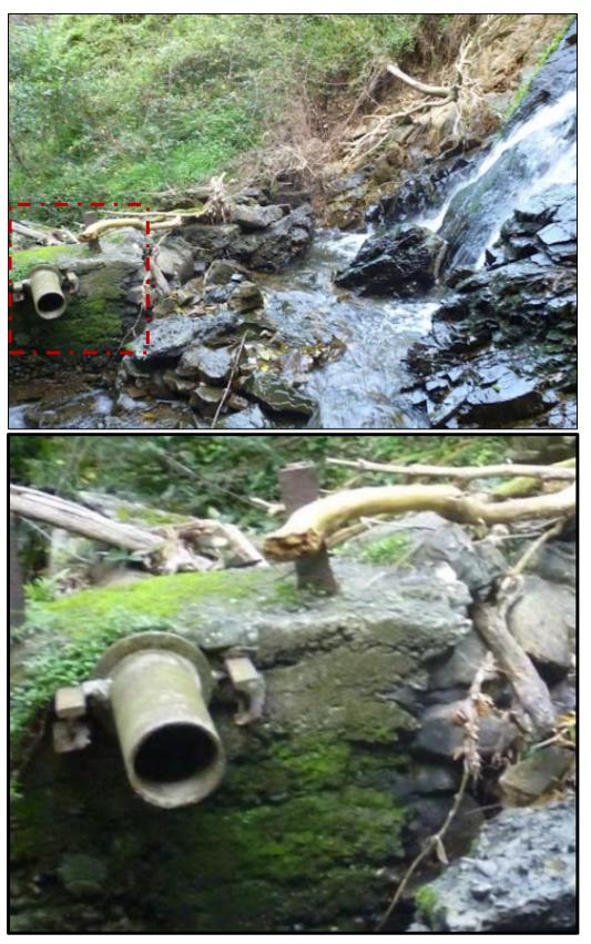
View of stream. Note on far left of image is stonework covered in a layer of concrete. During the nineteenth century, stone dams were sometimes covered in a layer of concrete for protection (Cadenhead, 2023; Greater Wellington Regional Council, 2007).
