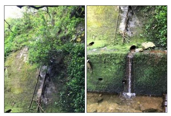
An acees ladder tuns up the dam and pipes set into the dam help drain water (Daubé & Wellington City Council, 2022).
