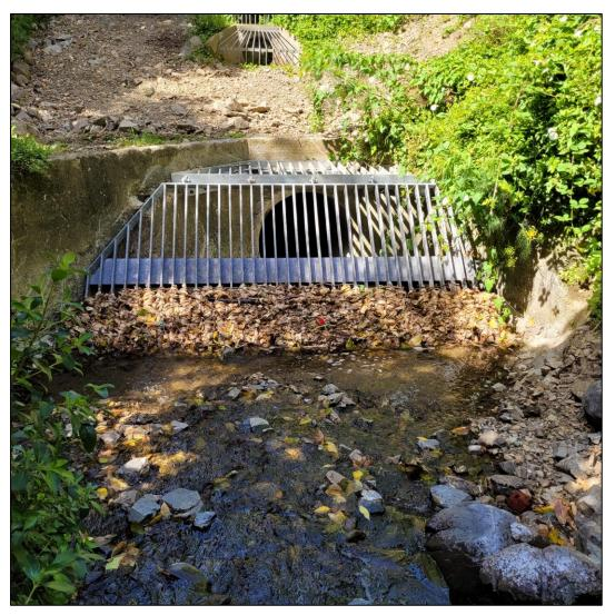
View of Tyers Stream culvert with new grill (Cadenhead, 2023).
