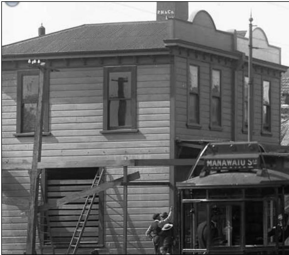
Detail from “Intersection of Riddiford Street, Mansfield Streets and Russell Terrace, in Newtown, Wellington”. Note the small wooden verandah over the shop entrance. A large square opening in the Rhodes Street elevation seems to be in the process of being boarded up (S. C. Smith, 1910)
