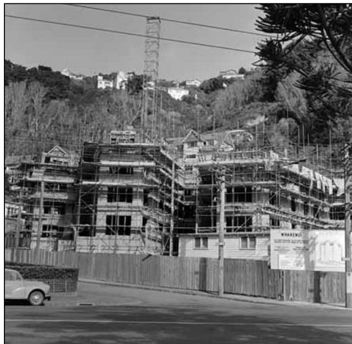
Apartments being built, Oriental Bay, EP/1958/3116-F, Alexander Turnbull Library.
