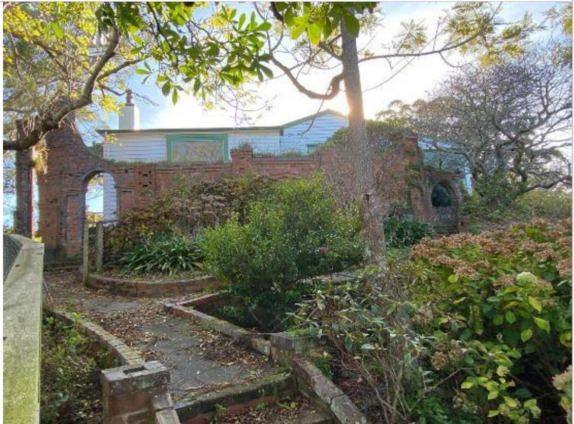
Figure 72. Walls about house from south. Note detailed brick work, with ledges, arches, contrast colours, projections and recesses, and openings for plants. The brick work is of considerable height in places. The moon gate to the right of this image is now fenced off.
