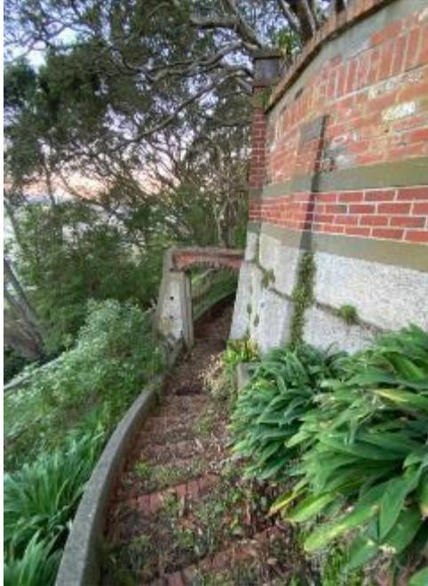
Figure 56. View from steps down behind semi-circular viewing platform. Note arch and contrasts between brick and concrete and plaster.
