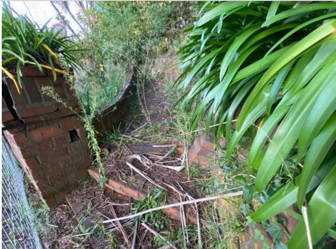
*Figure 16. The bottom of path – brick risers and concrete treads. Brick retaining wall to RHS.*
