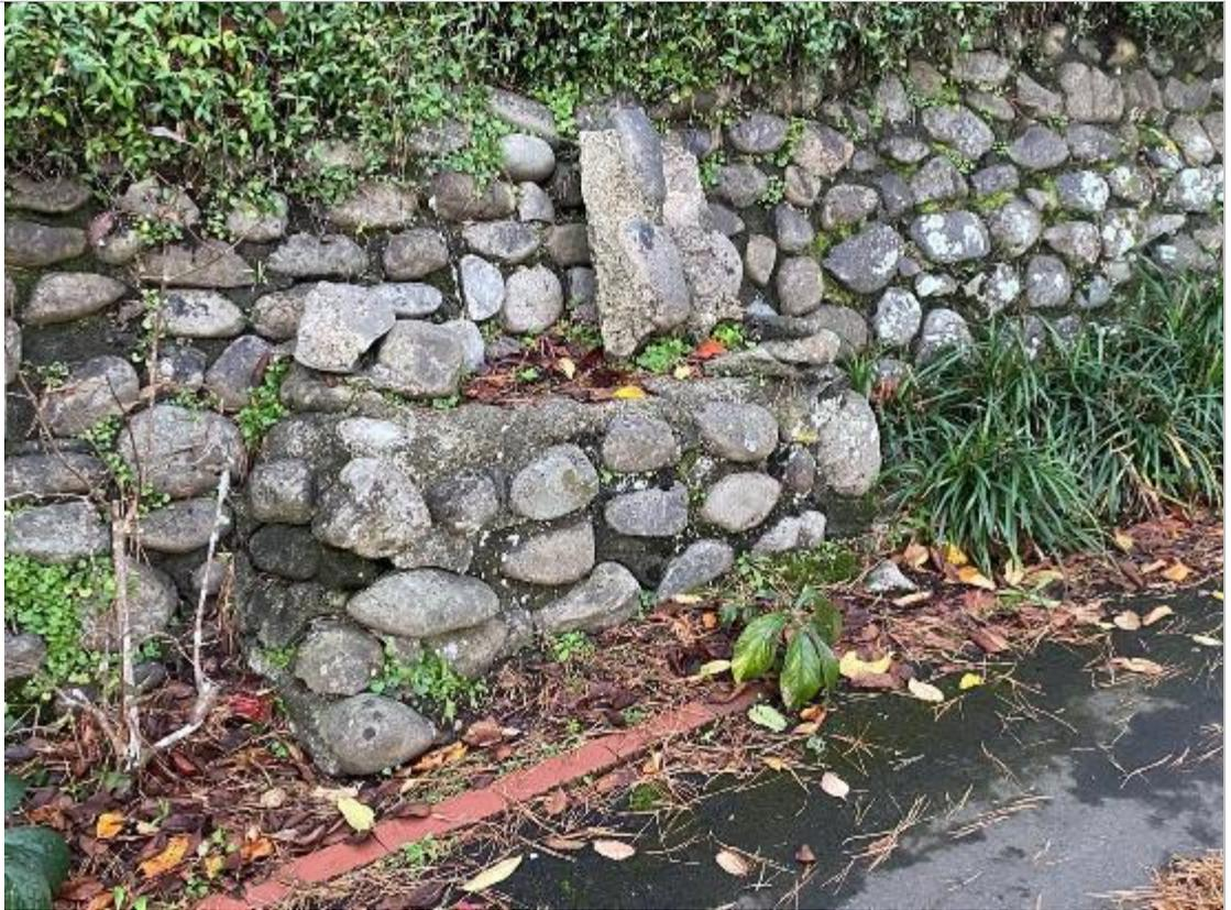
Figure 61. Seat formed in the random stone retaining wall between the two groups of piers on the 'down loop' drive.
