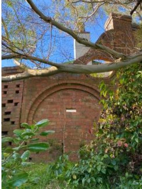
*Figure 73. Filled in arch in wall at west. Note perforations - possibly for planting.*
