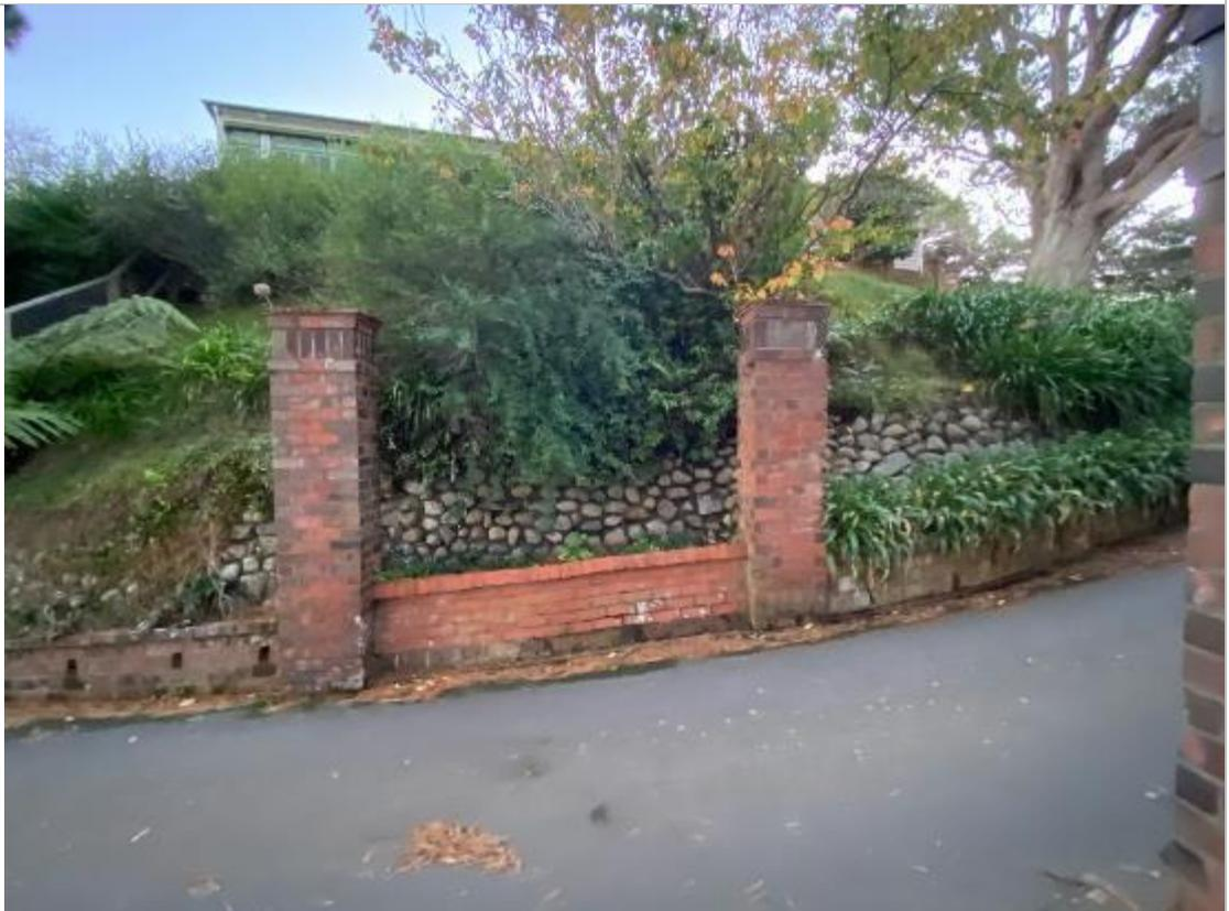
*Figure 50. The western piers in the upper group of four piers on the 'down loop' driveway. Note the brick kerb, brick low retaining wall, the random stone upper retaining wall, and the house above.*
