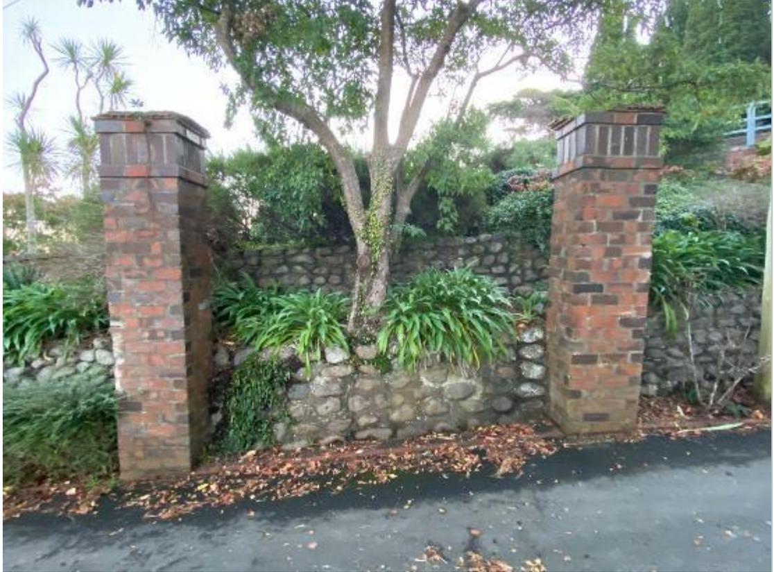
*Figure 63. Internal view of the lower group of piers on the 'down loop' drive. Note that there are random rock retaining walls between the piers in this location instead of the brick elsewhere.*
