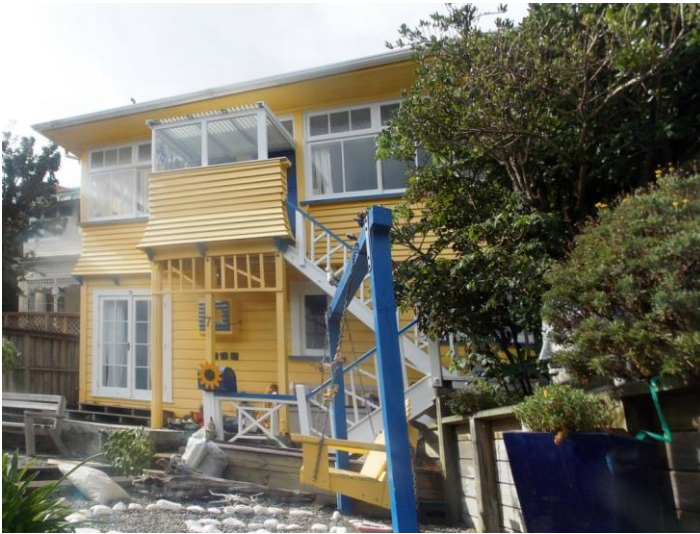
Image: 7 McIntyre Avenue, M. Kelly 2016.
