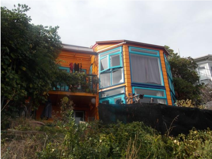
Image: 5 McIntyre Avenue, M. Kelly 2016.
