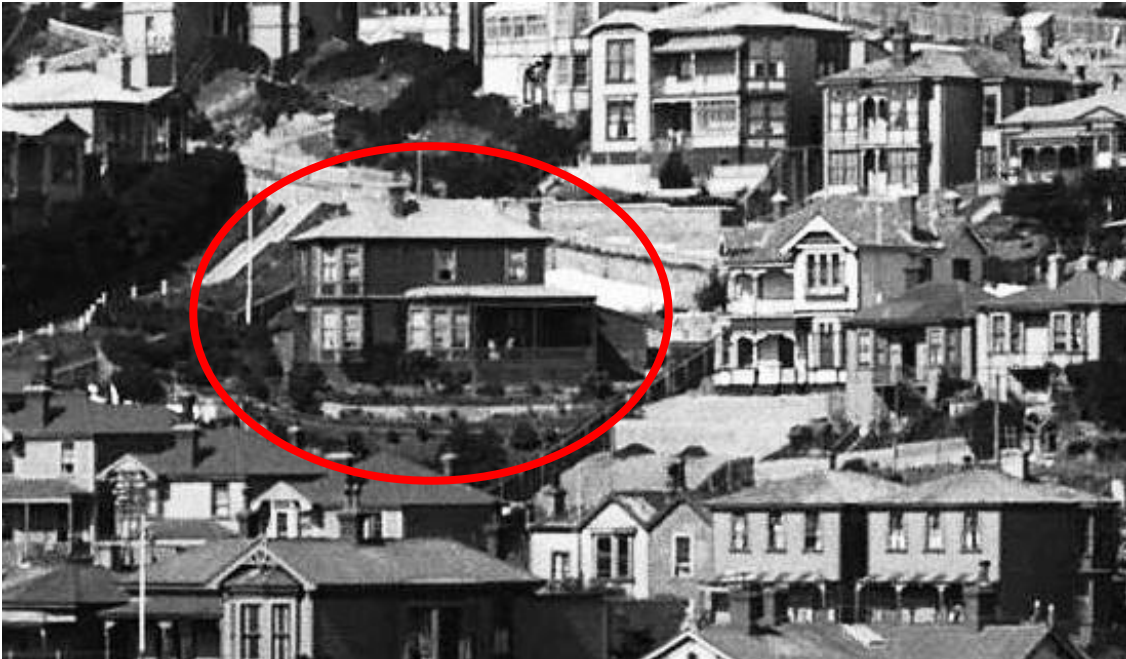
No. 2 Kennedy Street is in the middle of this image, taken about 1910, facing the other way from the rest of the houses around it. Prior to 1935 the verandah wing was only single storey. (S.C. Smith, 1/1-022832-G, Alexander Turnbull Library).
