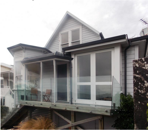
Image: 15 McIntyre Avenue, M. Kelly 2016.
