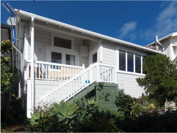
Image: 13 McIntyre Avenue, M. Kelly 2016.
