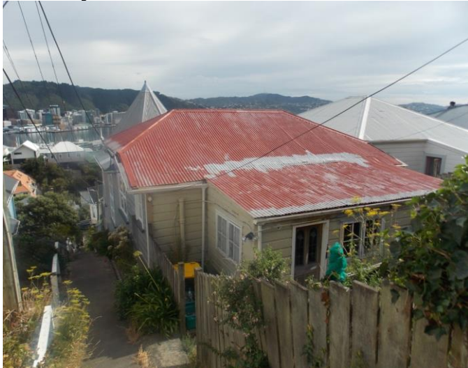
Image: 1 McIntyre Avenue, M. Kelly 2016.
