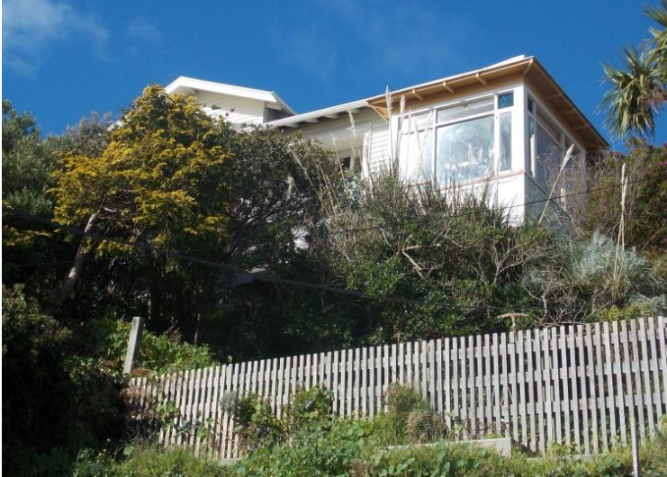
Image: 11 McIntyre Avenue, M. Kelly 2016.
