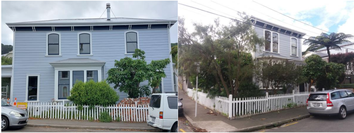
Image (left): Albany Avenue elevation, WCC, 2022.
