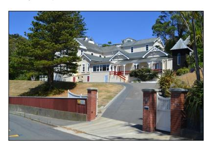
The original 1899 School House and Convent is still recognisable amongst the later additions and dormitories of the current complex. The original construction phase is seen in the main elevation upon site entry. It has low pitched gabled roofs and a wide verandah. There are sections of modern infill construction and a modern service ramp, however, the original elements are still clearly visible.
