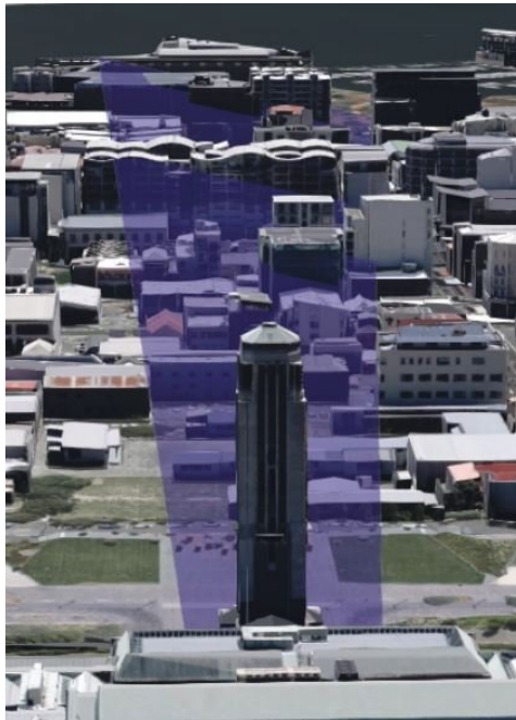
Figure 15: Showing existing development which has intruded into ODP-VS21.
