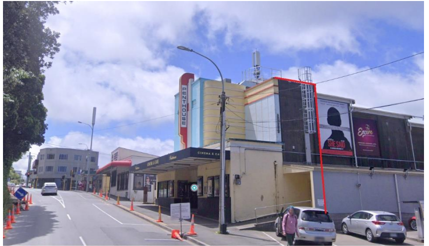
Figure 4: Extent of proposed listing looking north-east up Ohiro road
