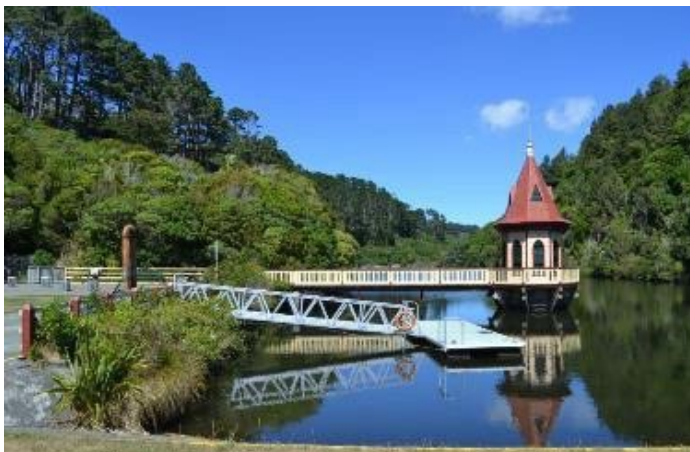
The Karori Reservoir Tower houses the valves that were originally used to control water levels in the Karori Dam. It is now part of the Zealandia Wildlife Sanctuary, and part of the story of water supply infrastructure in Wellington. (Photo: Wellington City Council, 2015)
