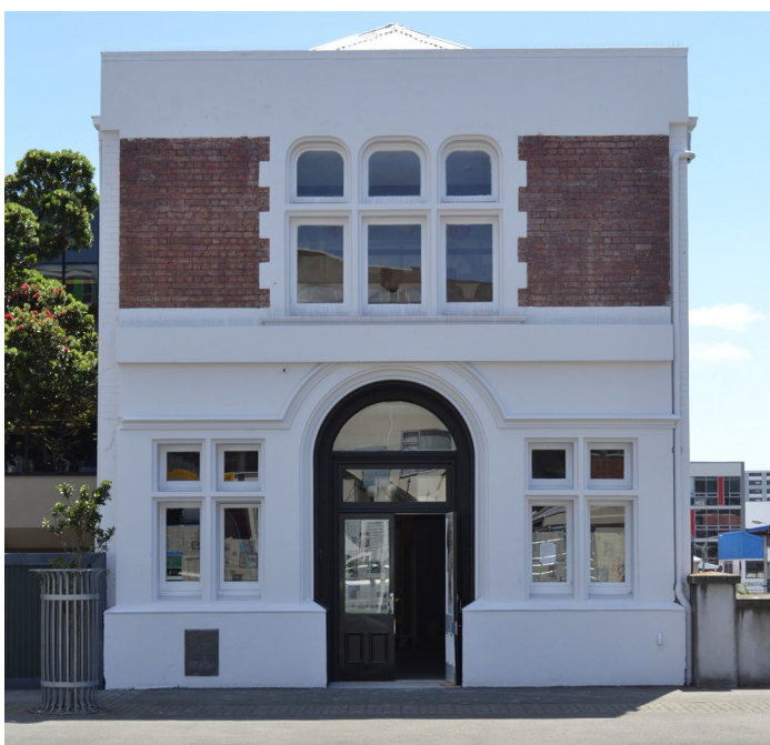
30 Arthur Street was relocated to allow for the construction of Karo Drive. It has been restored, strengthened and returned to a sustainable long-term use. (Photo: Wellington City Council, 2015)
