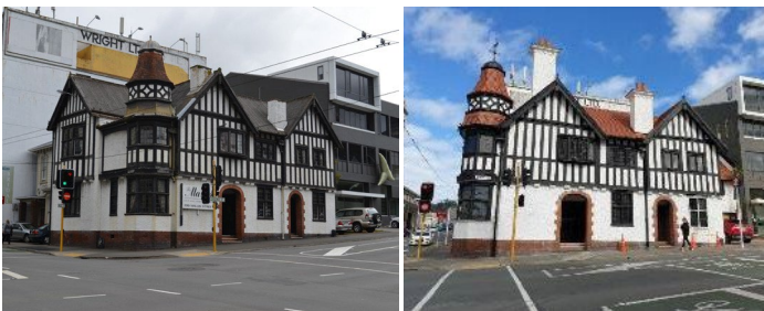
Parts of the chimneys at 200 Willis Street were removed in the early 20th century. The remaining unreinforced masonry above roof level was removed in c.2018, and the chimneys were reinstated in as lightweight replicas. The image to the left shows the building in previous years, the image to the right shows the completed works. (Photos: Wellington City Council (left 2015) (right 2021))
