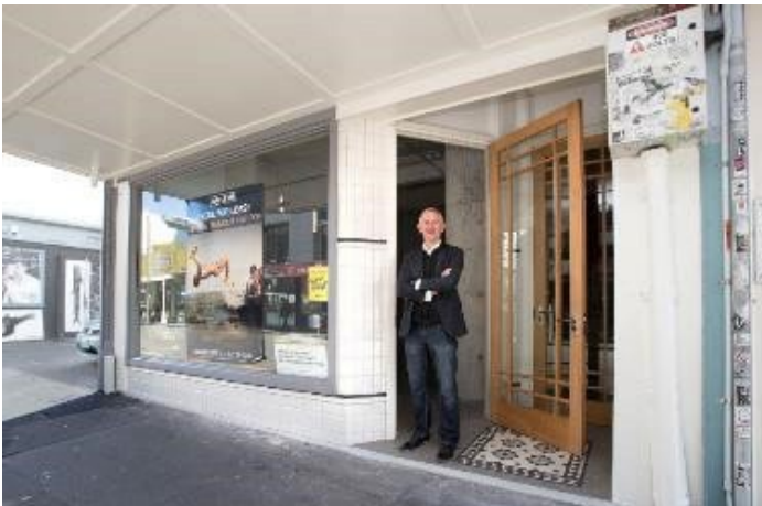
The new concrete moment-resisting frames installed at 216 Cuba Street ensure that the shop display window is not obscured. (Photos: Wellington City Council)
