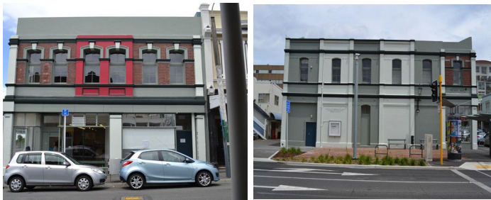
The Thistle Hall on Cuba Street is a good example of sympathetic works to strengthen a heritage building.
