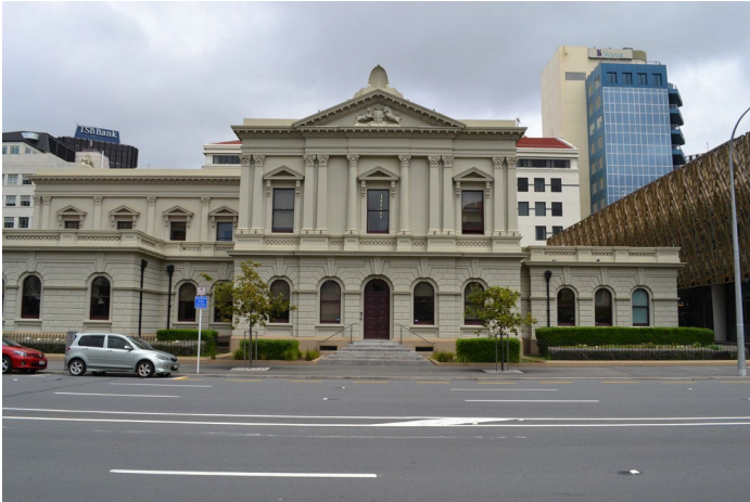
The former Supreme Court Building has been conserved and the pediment on the north elevation was reconstructed in 2009. (Photo: Wellington City Council, 2015)
