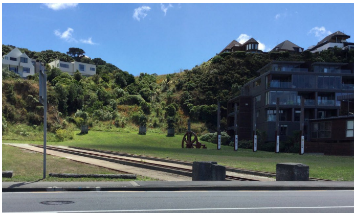
The Evans' Bay Patent Slip Heritage Area includes the slipway and equipment associated with early shipbuilding and repair. These have been conserved and the area is used as a public open space. (Photo: Wellington City Council, 2018)
