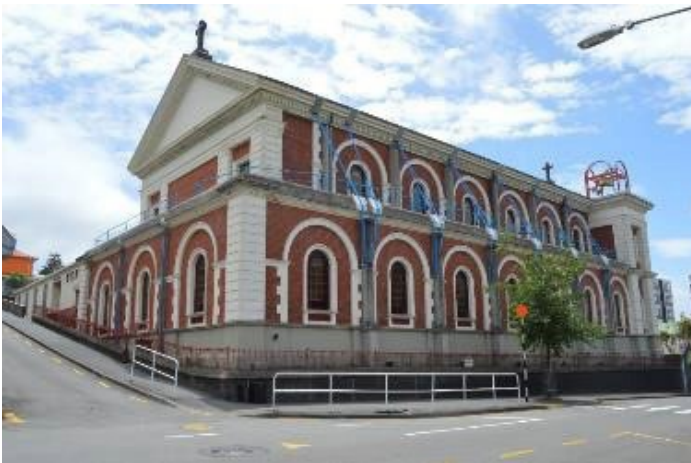
Temporary works at the Cathedral of the Sacred Heart on Hill Street. (Photo: Team Architects 2018)
