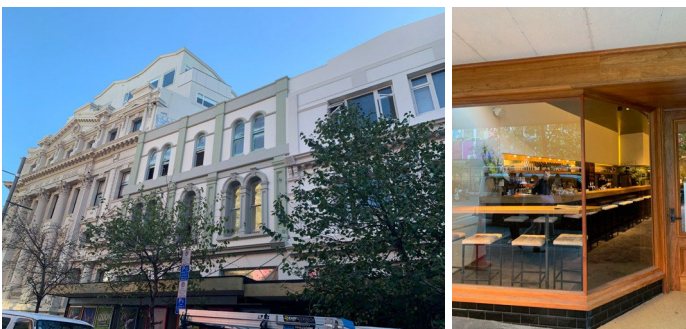
The restoration work undertaken at 54 Cuba Street has protected the heritage values of the Cuba Street Heritage Area, while adapting two buildings for sustainable long-term use. (Photos: Wellington City Council, 2019)
