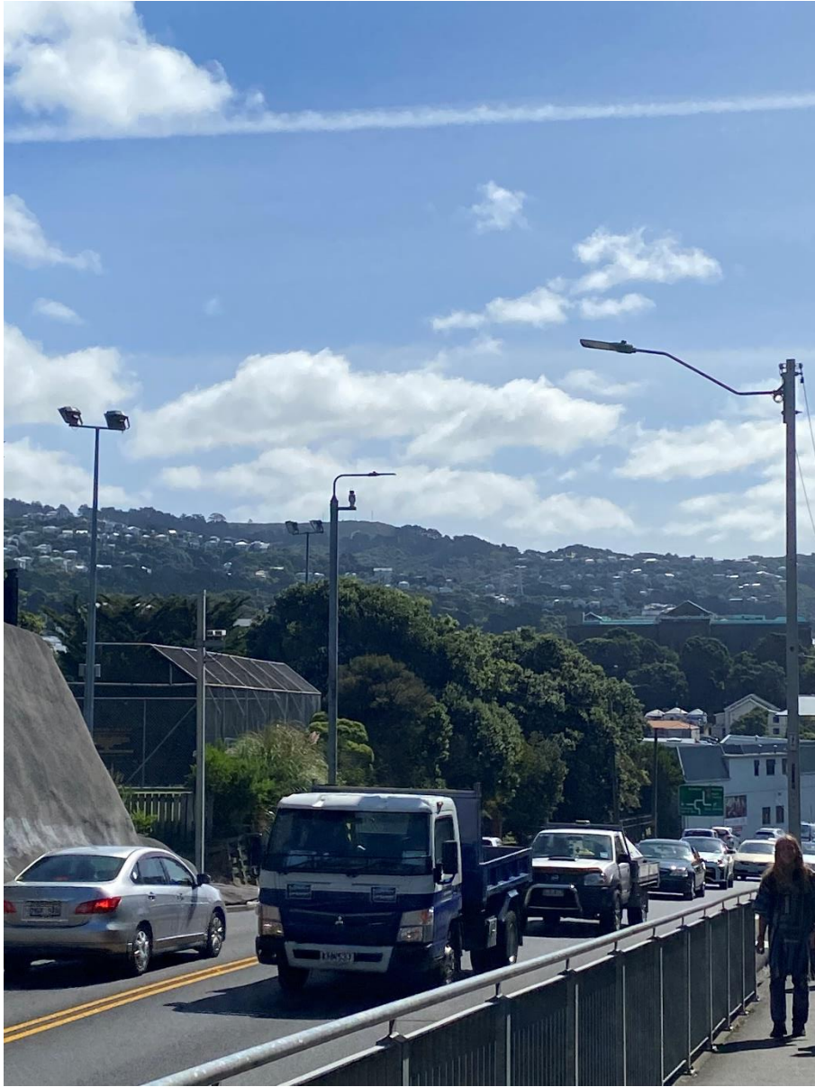
20 metres from portal – Brooklyn in view
