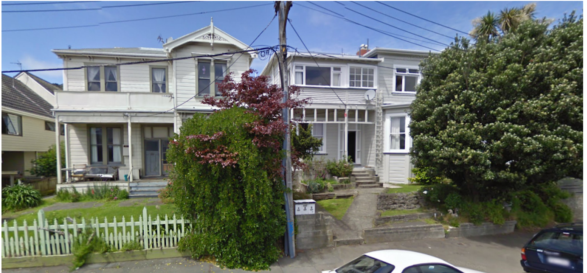
145 and 147 Brougham Street (noting that there has been vegetation growth since this photograph was taken, but no visible changes to the fabric of the buildings themselves).
