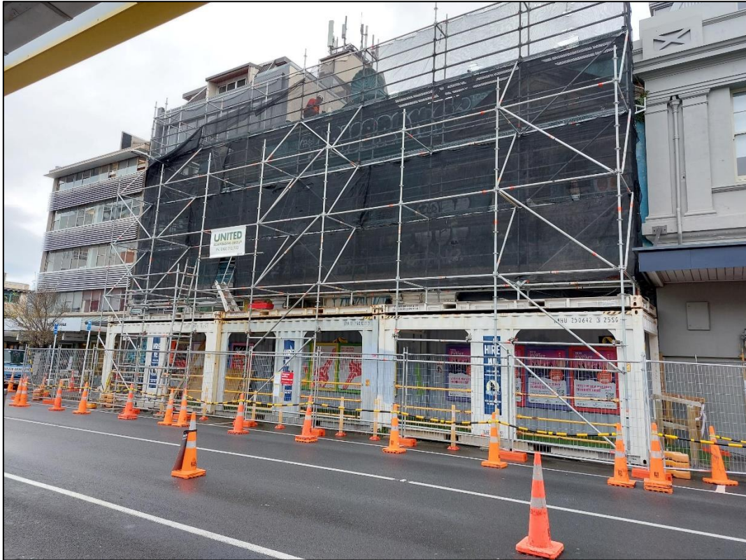
Figure 2: Image of demolition works looking south from Ghuznee Street
