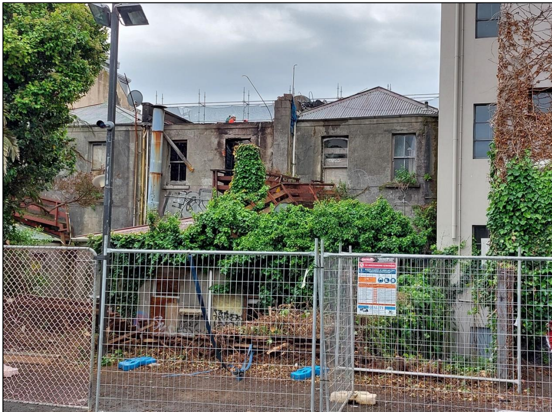
Figure 3: Image of demolition works looking north from Swan Lane
