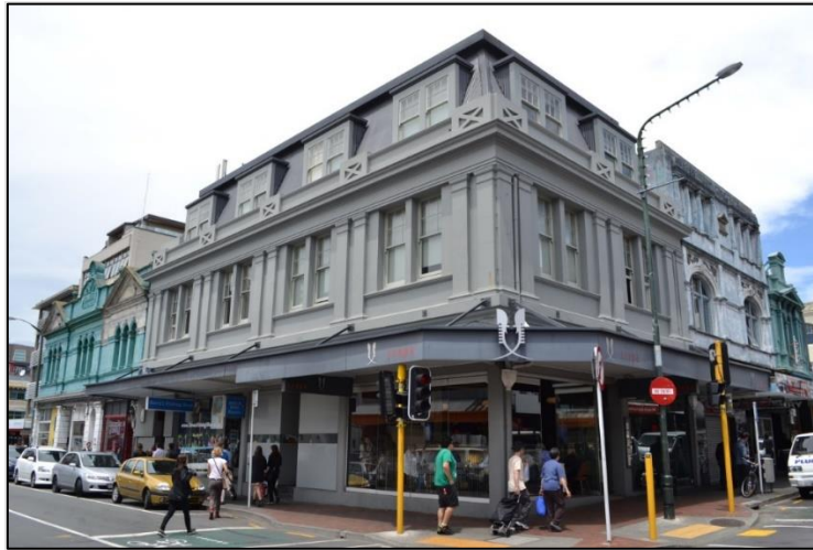
Figure 4: View of 43 Ghuznee Street (location of blue building) and 141 Cuba Street, viewed from Cuba Street. Credit: WCC
