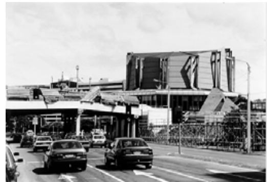
Landmark structures on entrance routes
