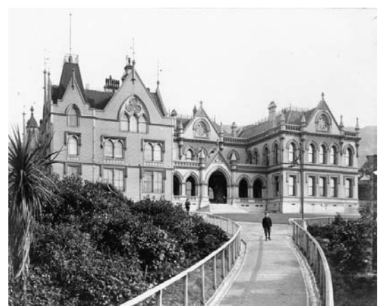
The Parliamentary Library after the completion of the 1899-1901 addition. The 1907 fire razed the earlier timber portion. (F106917½, ATL)
