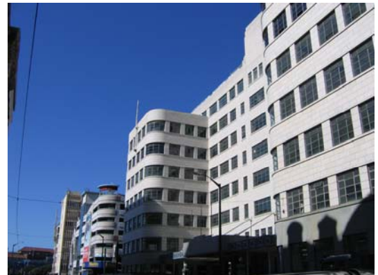
View north up Stout Street, showing the sight-line created by the parapet of the Departmental Building (in foreground)
