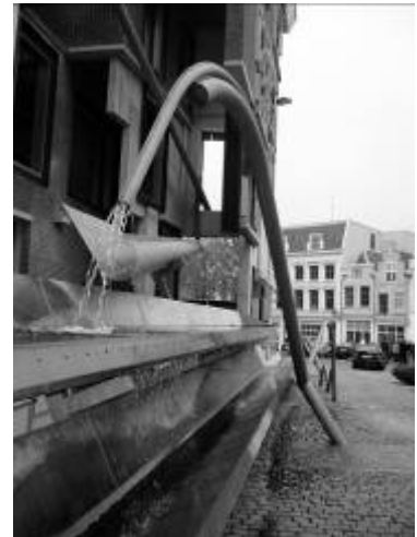
Richness of detail at ground level
