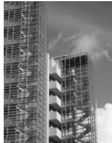
Sophisticated detailing in a contemporary building
