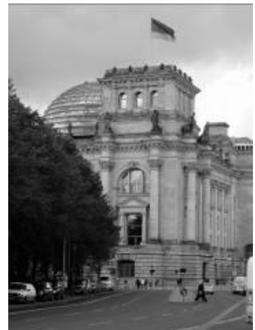
Publicly significant building demands contrast
