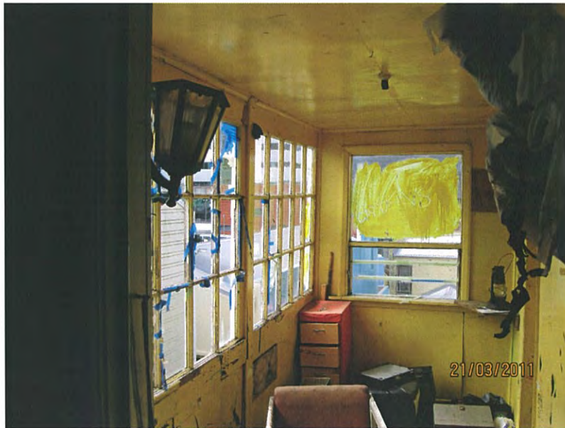
Figure 5: Closed in veranda, north elevation
