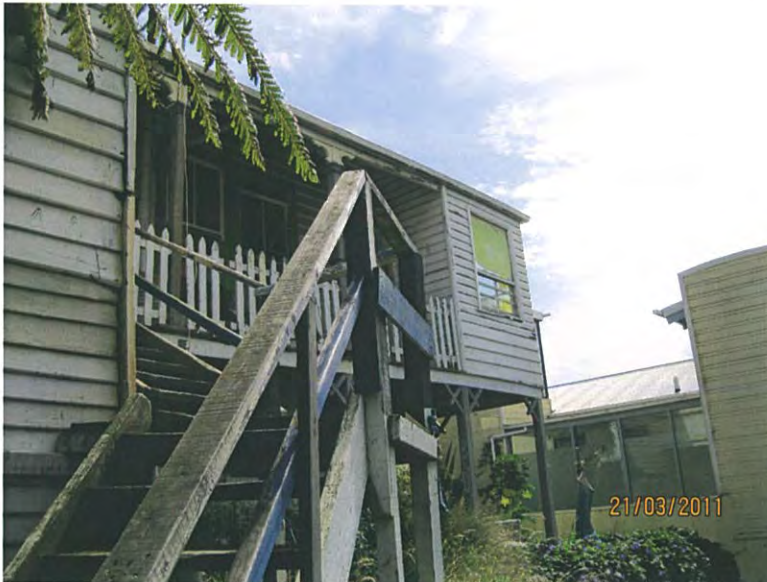
Figure 9: Stairs to east veranda
