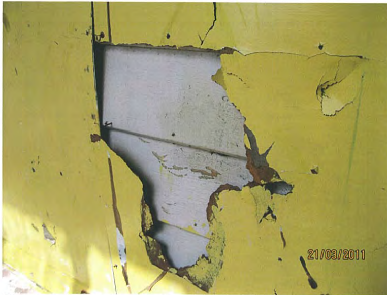
Figure 6: Original external weatherboards beneath cladding of north veranda
