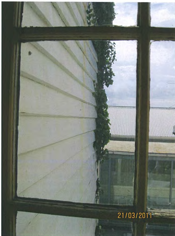
Figure 7: Weatherboards on front (east) elevation
