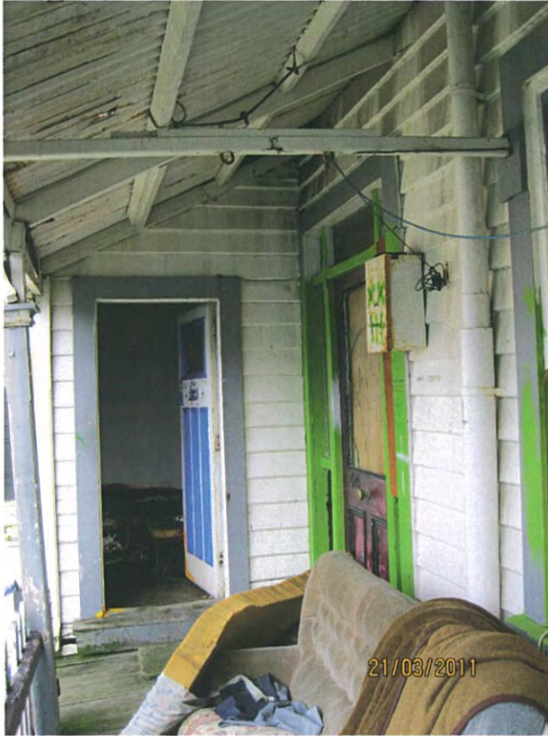
Figure 4: Front (east) veranda
