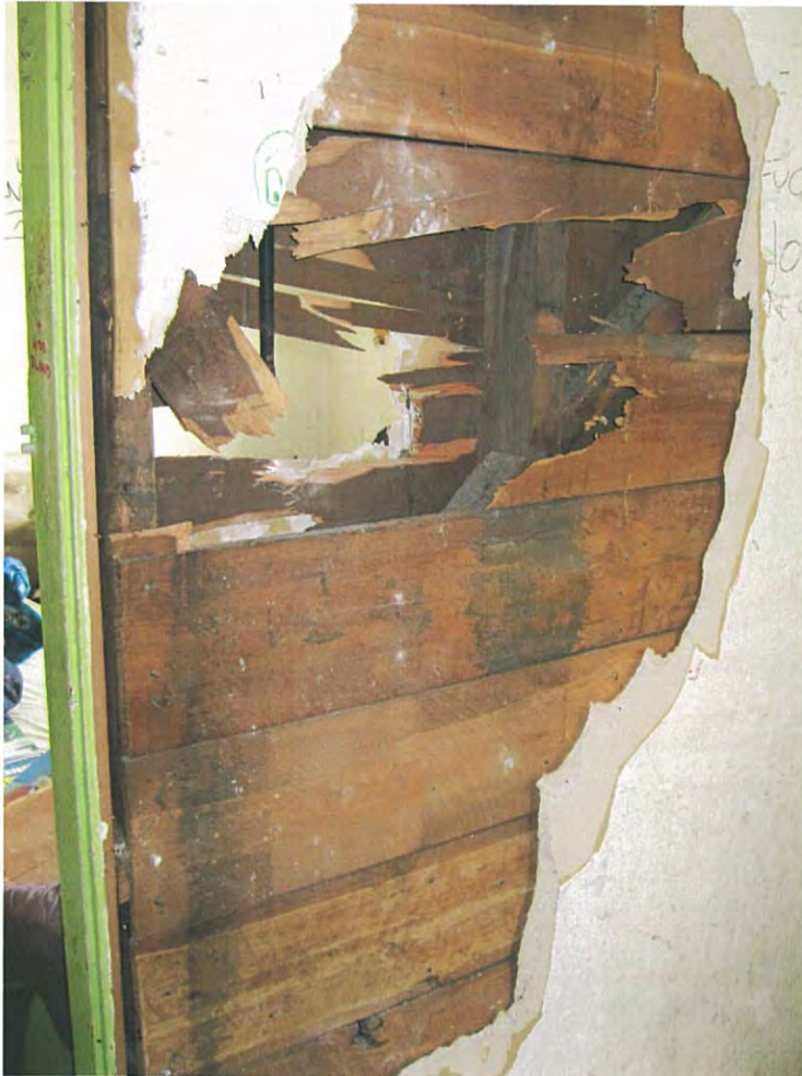
Figure 10: Sarking beneath plasterboard
