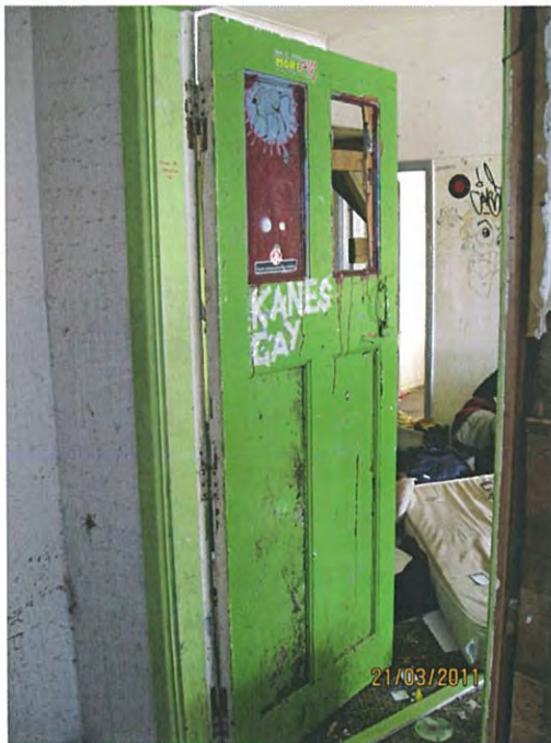
Figure 12: Possible exterior door reused in interior
