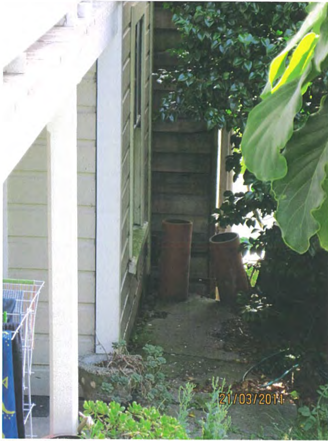
Figure 8: Weatherboards on south-east corner of house, seen in centre of picture past closely adjacent neighbouring house
