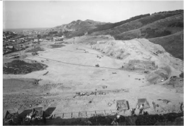
**Figure 4: Hataitai Park under construction in 1932. Relief labour dug out banks and moved spoil in metal bins on rails.**
