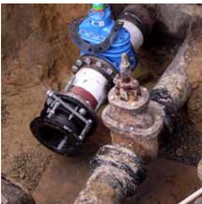
A new seismic coupling is fitted to a water main.
