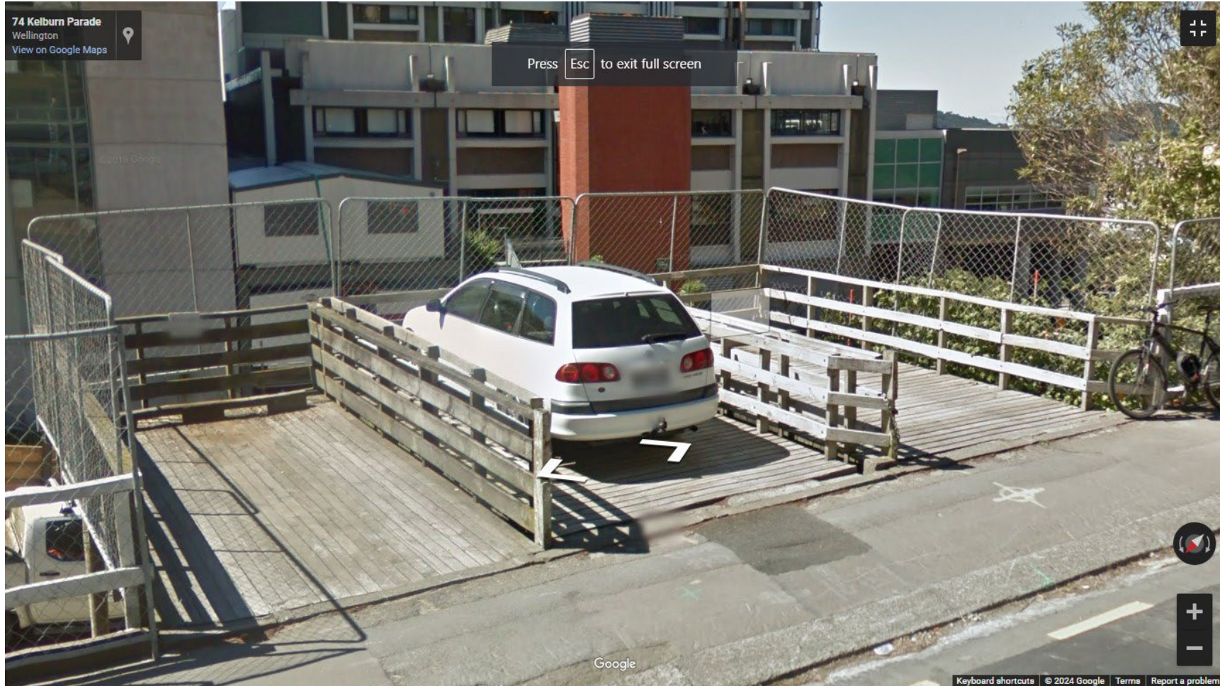
Kelburn Parade car decks before being demolished
