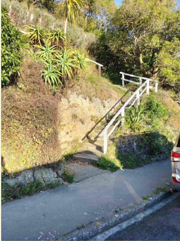
Lower Access stairs
