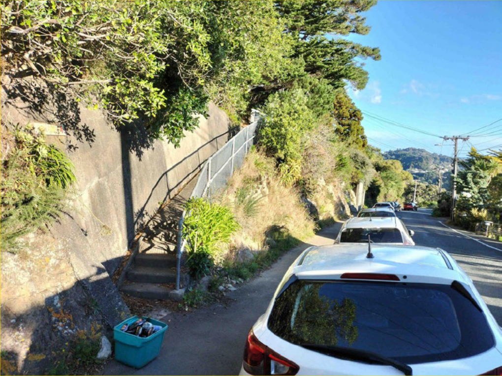
Upper Access point
