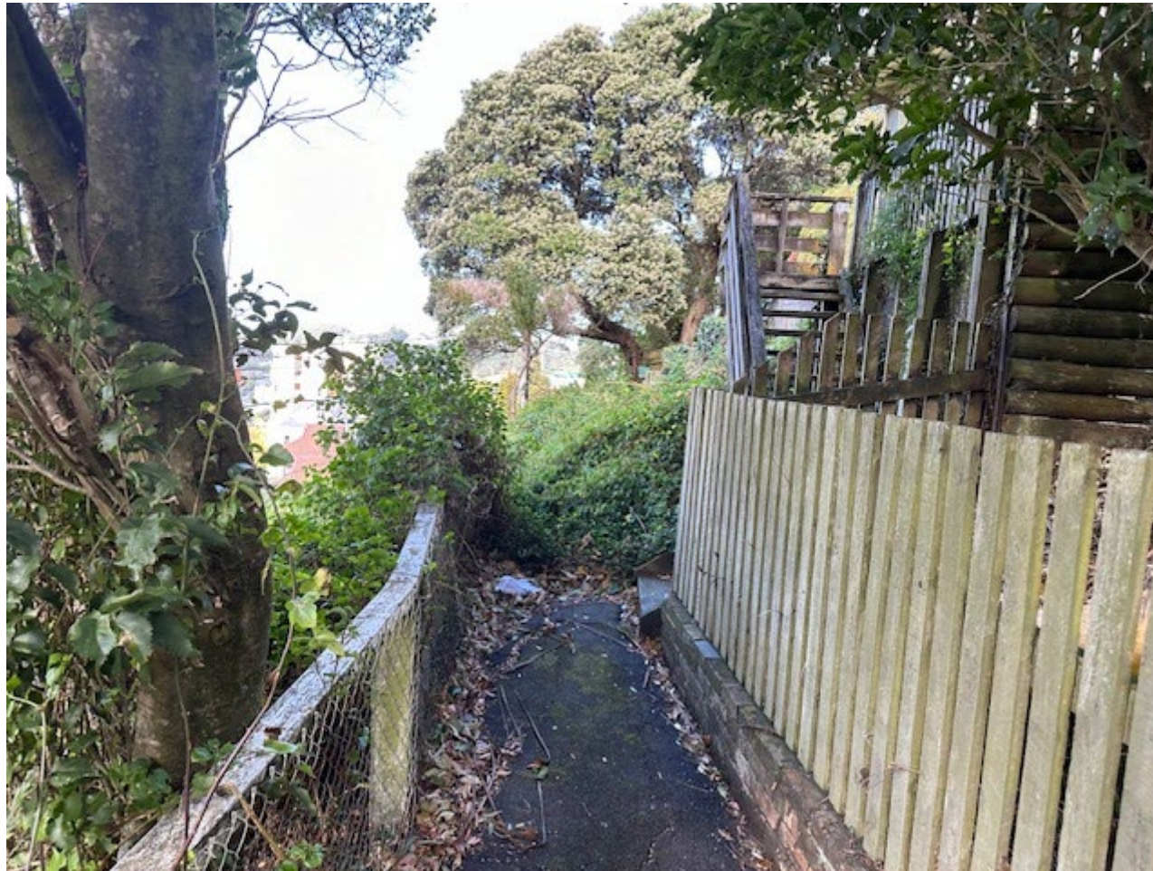
Previous thoroughfare path blocked by dumped excavated earth obstructing egress in emergency at 76KP
