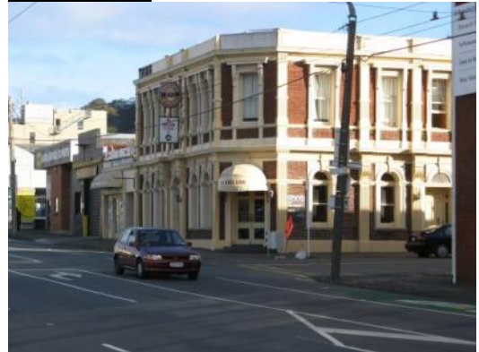
One of the few dispersed heritage buildings, contributing positively to the streetscape
