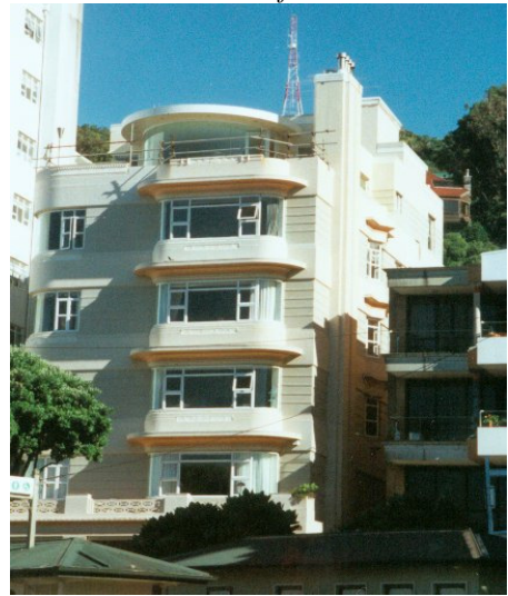
Façade features and detail on side elevations
