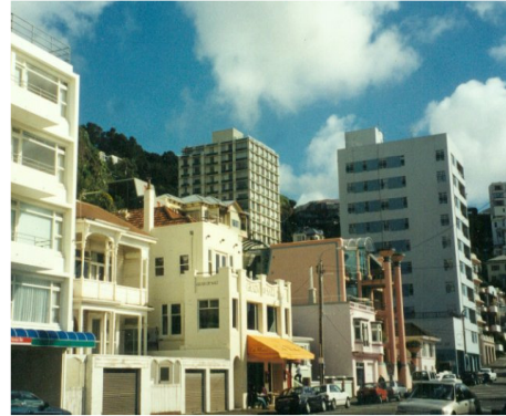
Side elevations visible from the street
