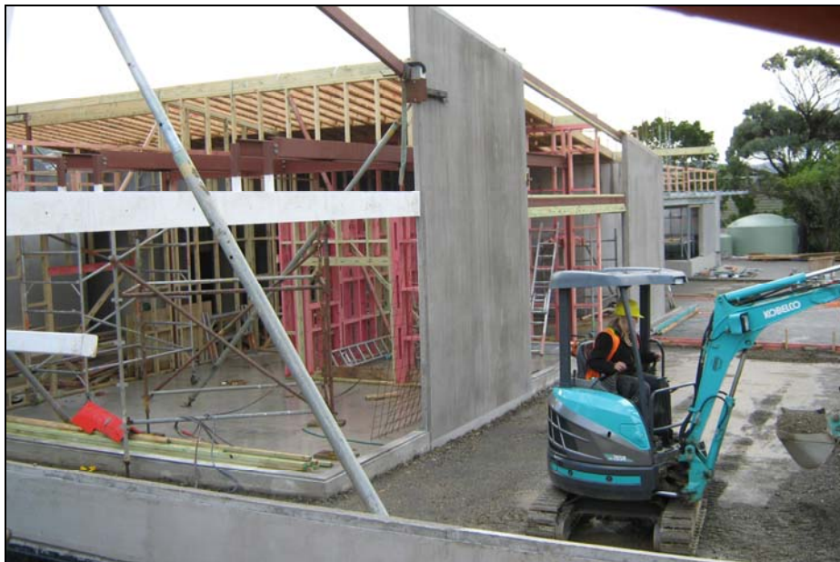
Construction progress on The Nest, May 2009
