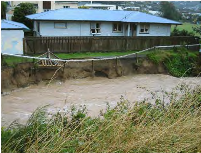
Porirua Stream 13 Tawa St. Erosion 16 Feb. 04
