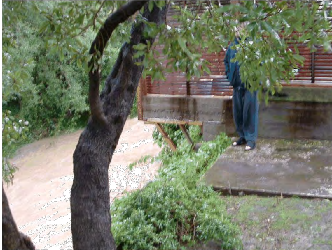
Deck 24 Oxford Street over Porirua Stream 17 Feb 04 – 7 yr return period flood event on the Porirua Stream
