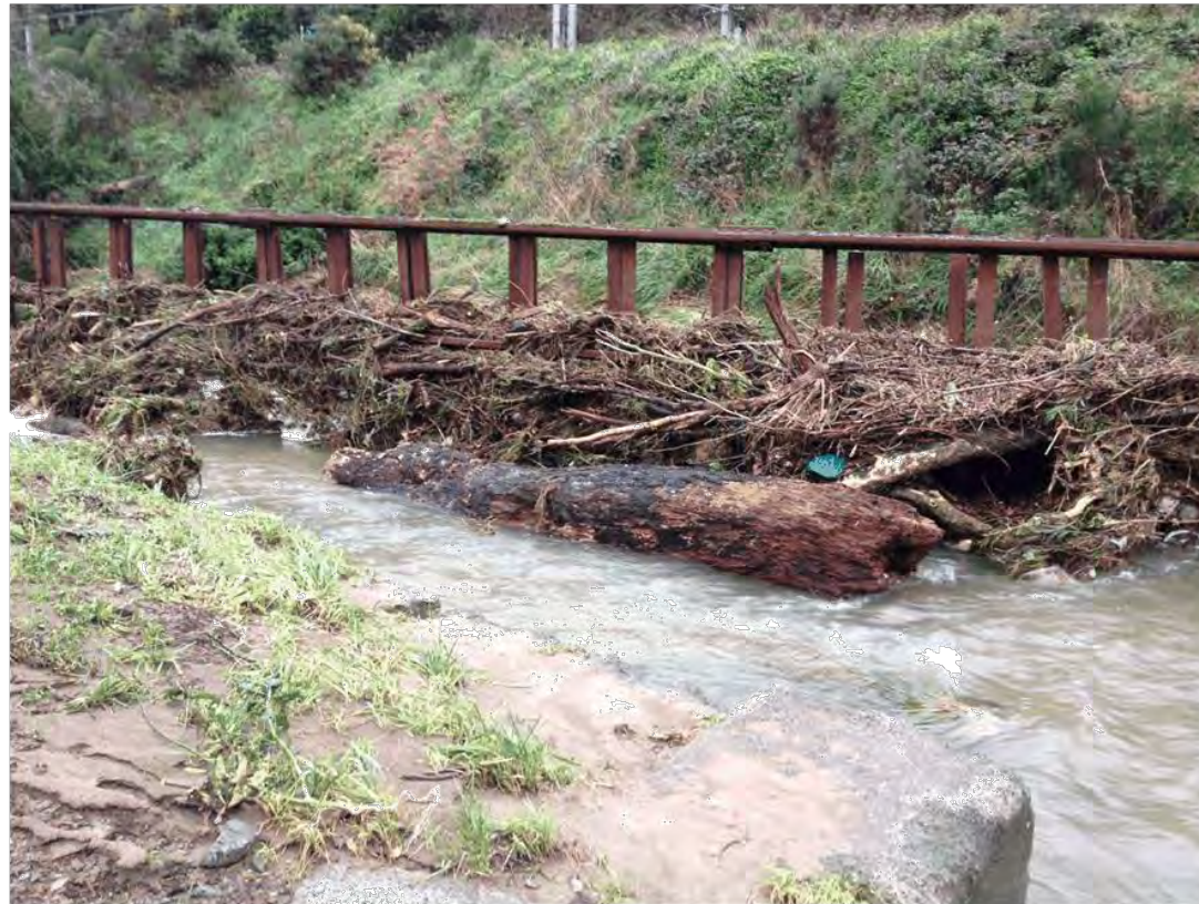
Glenside Debris Arrester
