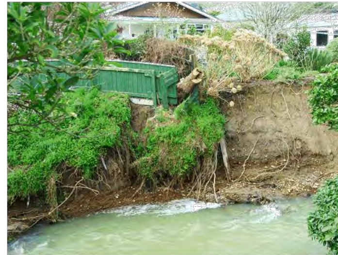
Porirua Stream - Linden Erosion. 4 August 2006
