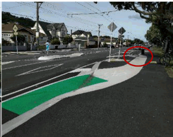
Figure 2-6: Photo showing green coloured cycleway markings provided on departure only. Note also the cycle symbol in advance of the green surfacing blending into the concrete surface
