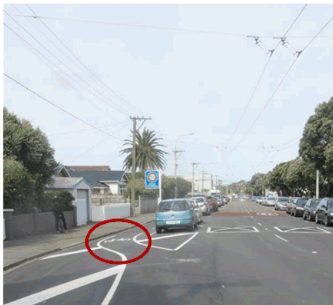
Figure 2-5: Photo showing a lack of green coloured cycleway markings on diverge from the "sharrow" lane into the cycleway
