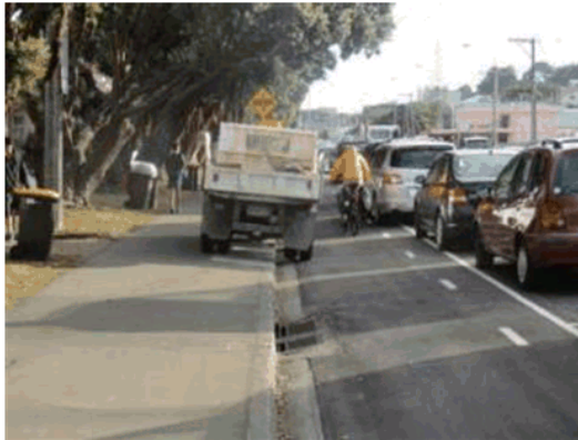
Figure 2-14: Photo showing a combination of vehicles parked across the buffer zone and on the footpath, limiting the width available to the cyclist
