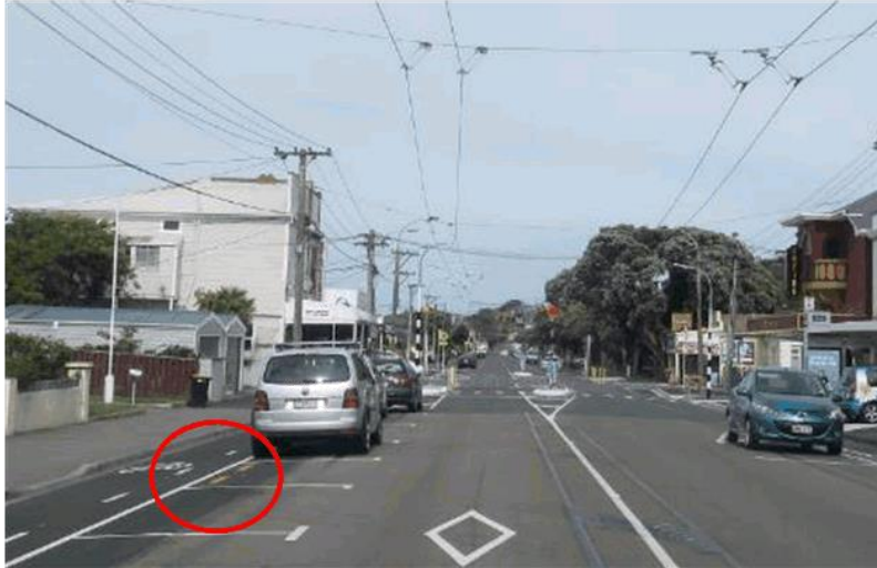
Figure 2-31: Photo showing no-parking line marking between parking spaces, north of Mersey St
