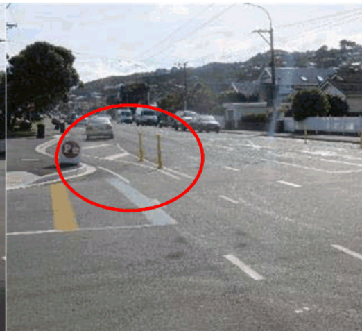
Figure 2-22: Photo showing the safe-hit posts installed at the western side of the Humber St intersection
