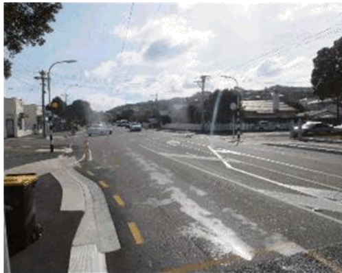
Figure 2-1: Photo showing ghost right turn bay markings
