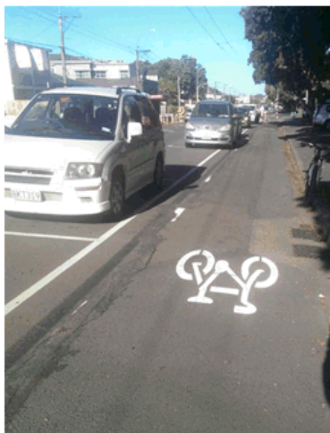
Figure 2: Buffer Zone marking poor condition
