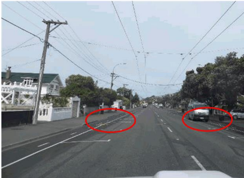
Figure 2-32: Photo showing a lack of no-parking line marking between larger parking spaces
