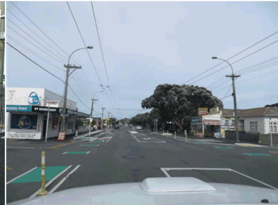
Figure 2-8: Photo showing green coloured surfacing across the Mersey St intersection, however there are no cycle symbols provided
