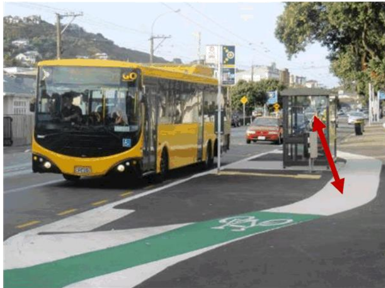
Figure 2-13: Photo showing a clear bus stop shelter, north of Avon St, providing good intervisibility between modes
