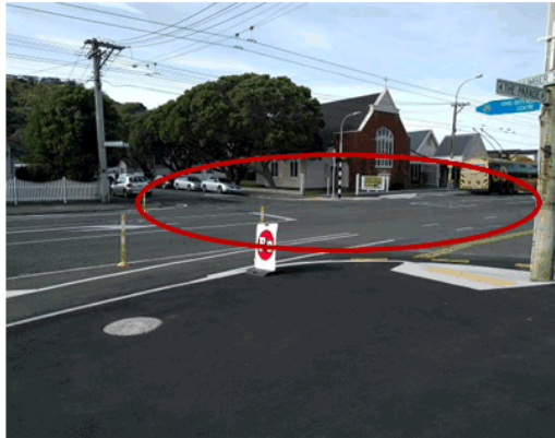
Figure 2-7: Photo showing a lack of green coloured surfacing and cycle symbols across the Humber St Intersection
