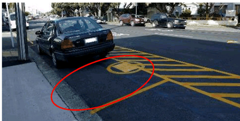
Figure 2-29: Photo showing the length of the southern disabled parking space (note the vehicle parked at the southern end of the space) and the fire hydrant located between the two parking spaces (currently located inside the southern disabled parking space), south of Medway Street
