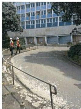
Figure 10. Looking along the entrance driveway leading to the eastern aspect of the Gordon Wilson building. (Archifac-Architecture & Conservation Ltd., 2014).
