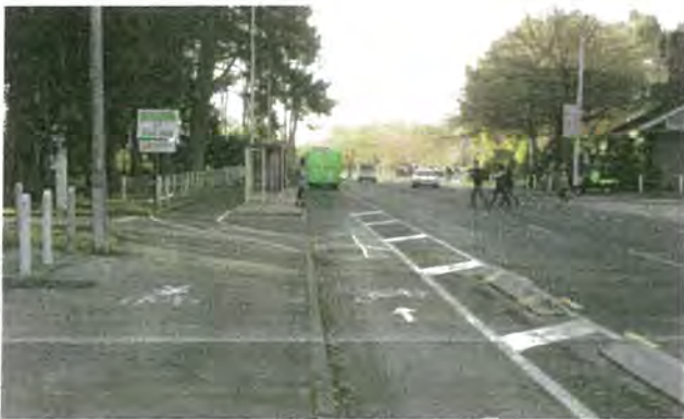
Bus stop bypass with a shared footpath. Photo: Glen Koorey (cyclingchristchurch.co.nz)
