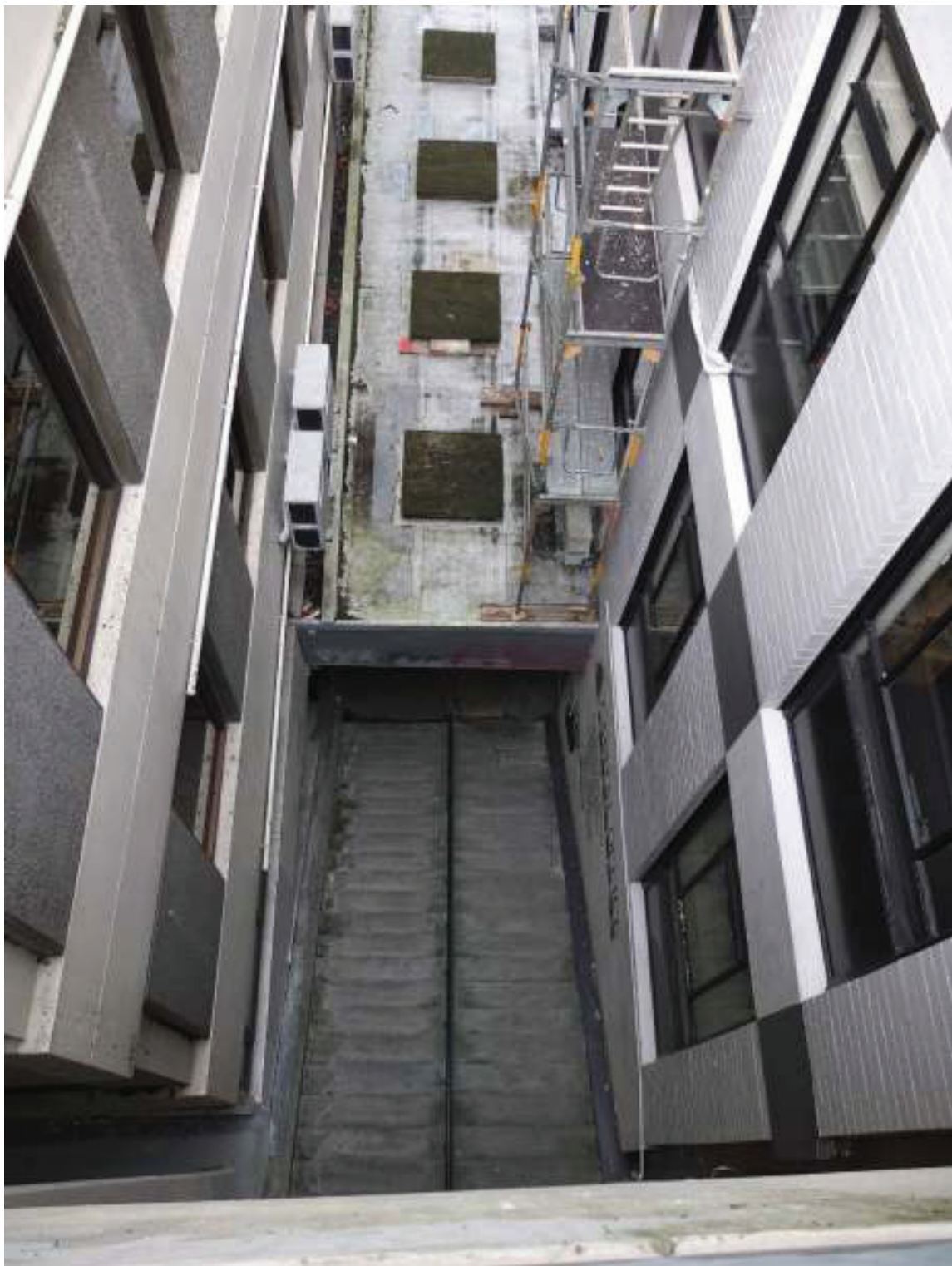
13 another view of broken down old canopy and plywood replacing Perspex also showing steps not protected from rain
