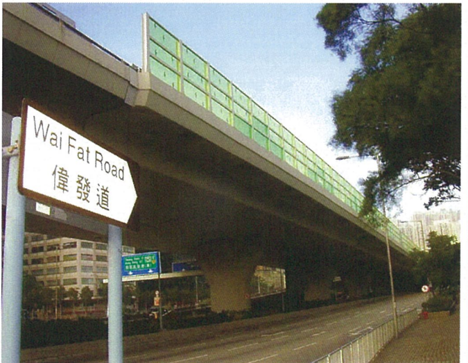
HK Wai Fat Street Kwun Tong Bypass Noise barrier
