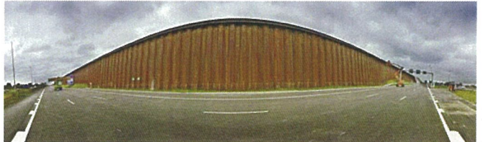
Noise barriers A2 motorway - Eindhoven | The Netherlands
