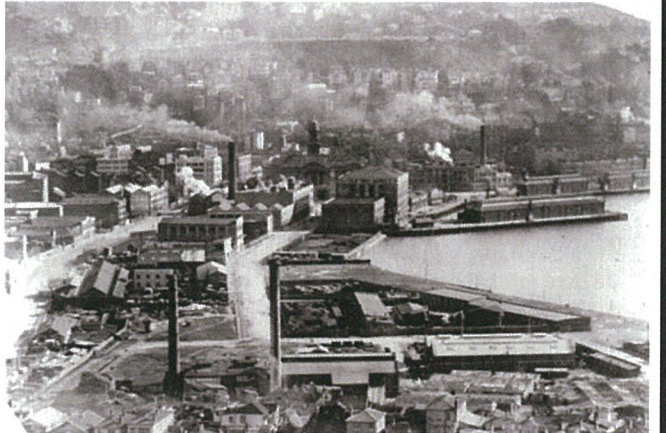
Fig 3: Before: City Destructor & WCC works depot
