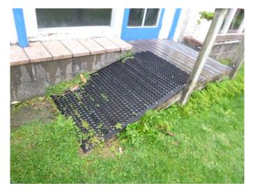
Example of none-compliant timber access ramps.
