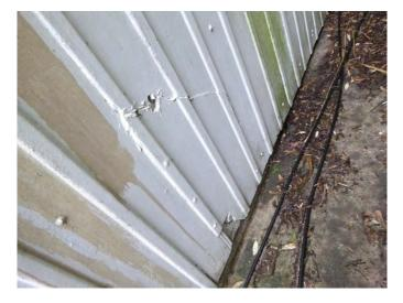
Historic damage and adhoc repair to suspected asbestos cladding on southern elevation.
