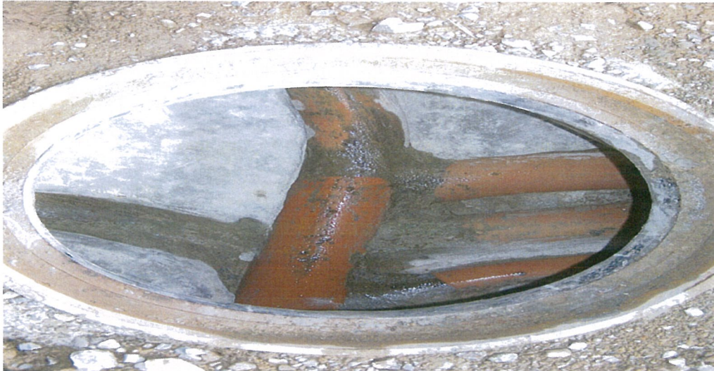
View 2 of manhole with subsoil drain connections
