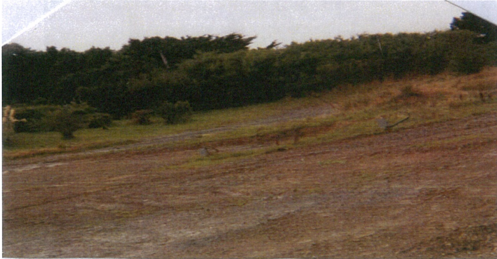
View of 101 - 109 Beazley Avenue site showing townhouses originally being built
