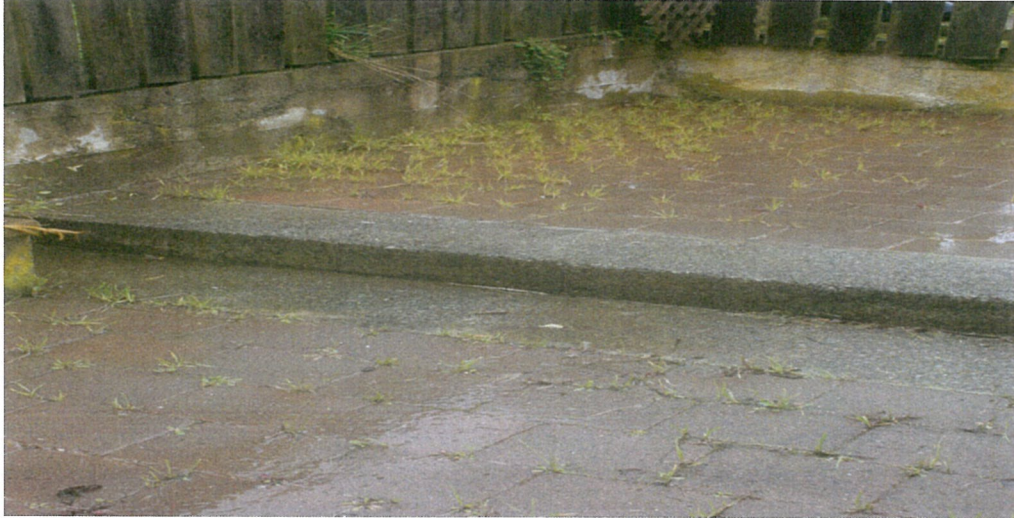
View 1 of manhole with subsoil drain connections
