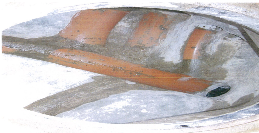
View 2 of manhole with subsoil drain connections
