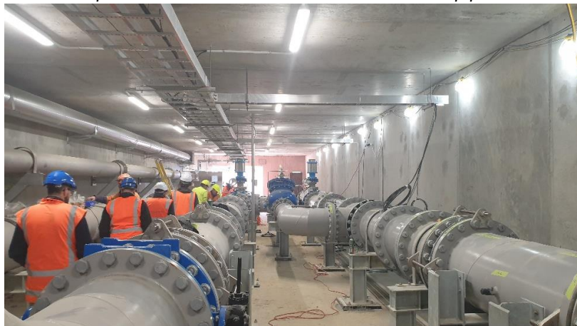
Completed reservoir structure and Access tunnel pipeline installation
