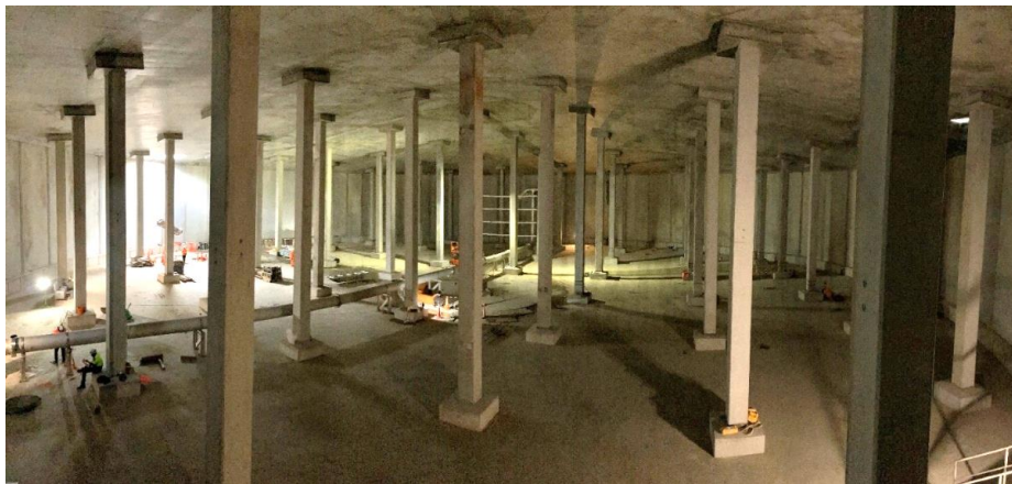
Completed reservoir structure and Access tunnel pipeline installation
