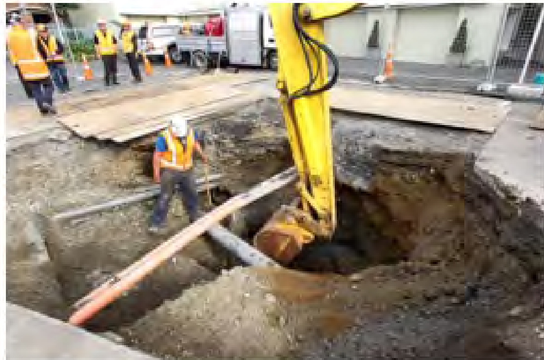
Sink hole in Hobson St – stormwater tunnel collapse
