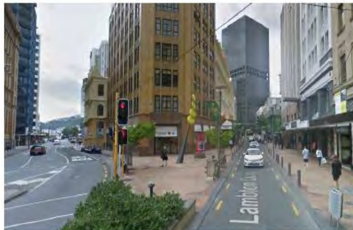
Figure 28: Old Bank Building
