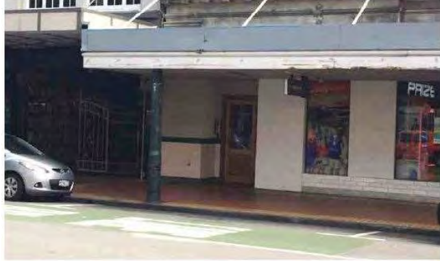
Figure 24 - Example of Unattractive Built Edge near Te Aro Park
