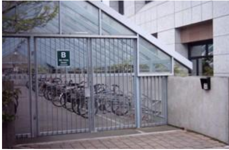
Figure 29: enclosure with swipe card access, electric gate, security cameras – Univ. of Canterbury (G. Koorey)
