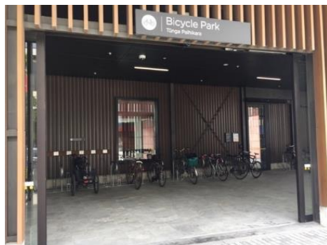
Figure 31: cycle parking with motorised sliding doors and e-bike charging, Christchurch bus exchange (J. Lieswyn)
