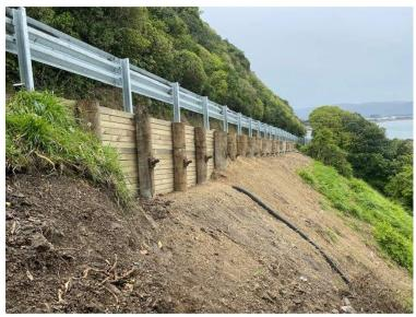
Figure 12 Horokiwi (anchored timber pole)
