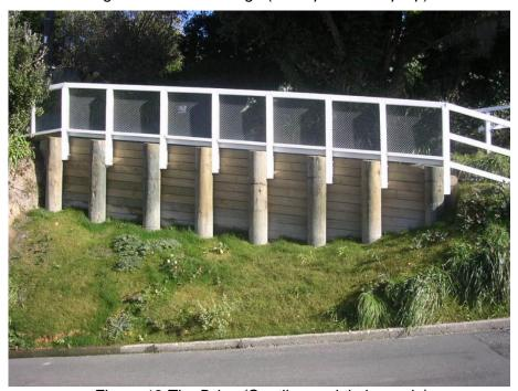
Figure 19 The Drive (Cantilevered timber pole)
