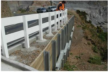
Figure 11 Horokiwi Rd (anchored steel pole)
