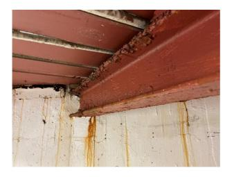
Significant corrosion roof beam Wakefield St pump station - WCC
