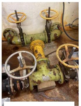
Pipe work in poor state -Featherston St pump station (PS08) -WCC
