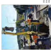
Workers lower shoring components into a trench for a project in Upper Hutt. The trench heights at which shoring must be in place have been reviewed by Welfington Water recently, to ensure workers performing tasks below ground level are safe.
